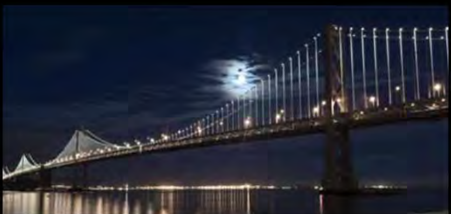
White LED Narrow Spots grazing down suspension hangers.
