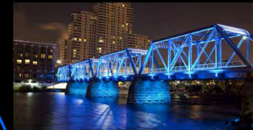
LED Color Changing floods tucked into corners of the truss structure.
