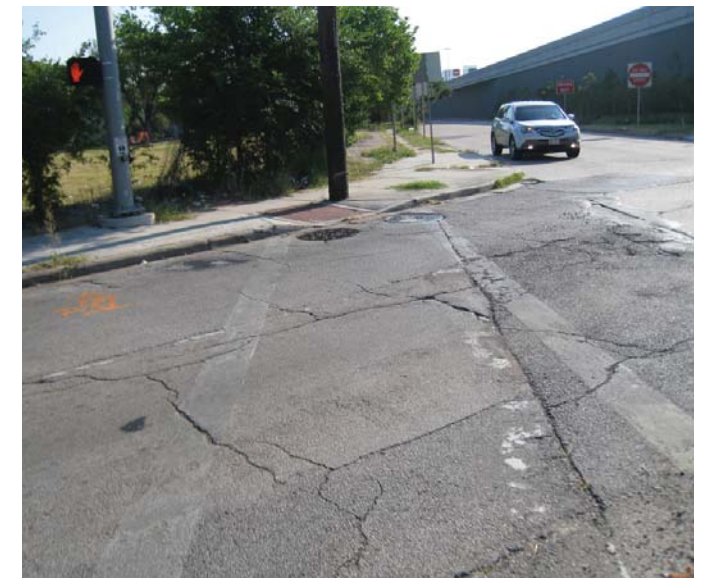
Photo 5-9, Segment 37 Richmond at Milam Multiple cracks , poor riding experience
