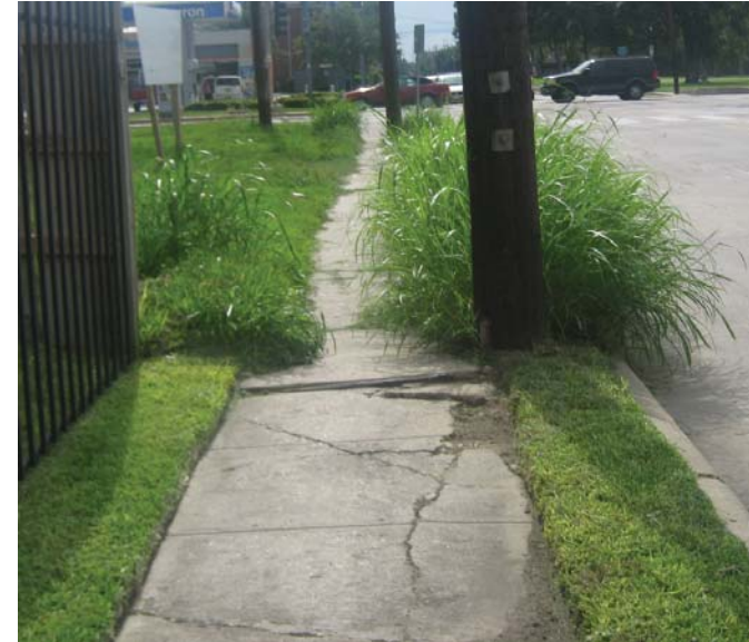
Photo 10-17, Segment 30B W. Dallas between Montrose and Columbus Cracking and overgrown vegetation
