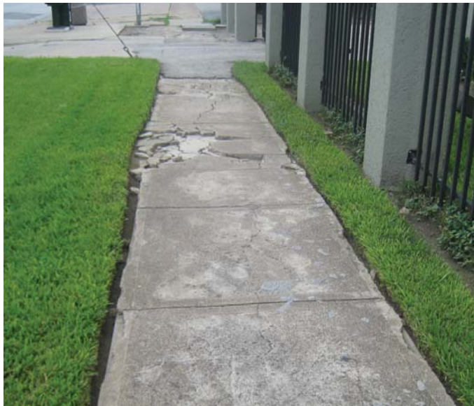
Photo 6-26, Segment 42B W. Alabama between Bute and Flora A section of the sidewalk has broken pieces which might create tripping hazards.
