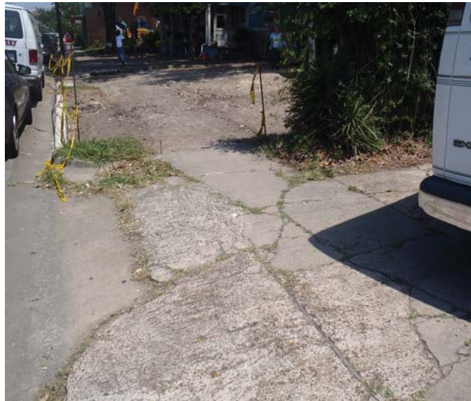
Photo 7-14, Segment 18B Westheimer between Elmen and Park Missing section of sidewalk
