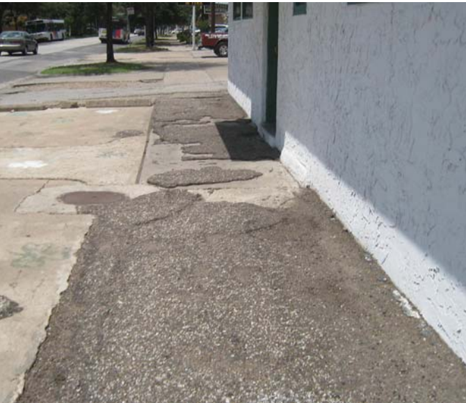
Photo 15-11, Segment 26B Shepherd between Indiana/Avalon and Fairview Asphalt over existing concrete is beginning to come up, creating possible tripping hazards.
