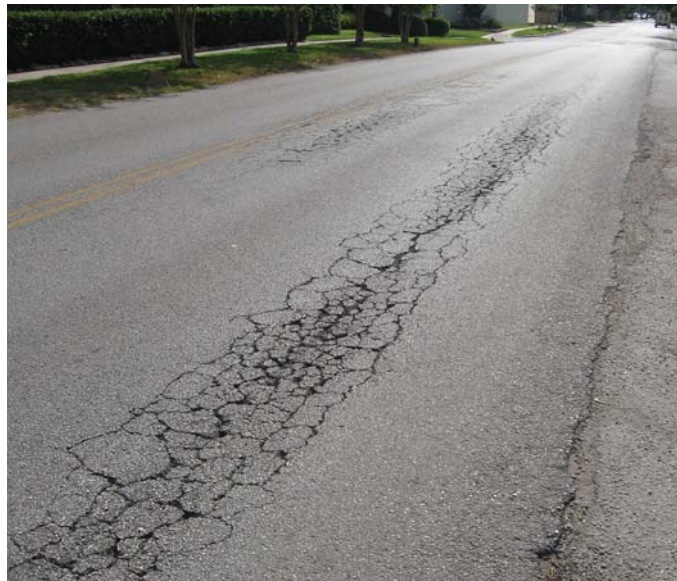
Photo 8-2, Segment 12B Fairview between Driscoll and Morse Alligator cracks where tires traditionally travel.
