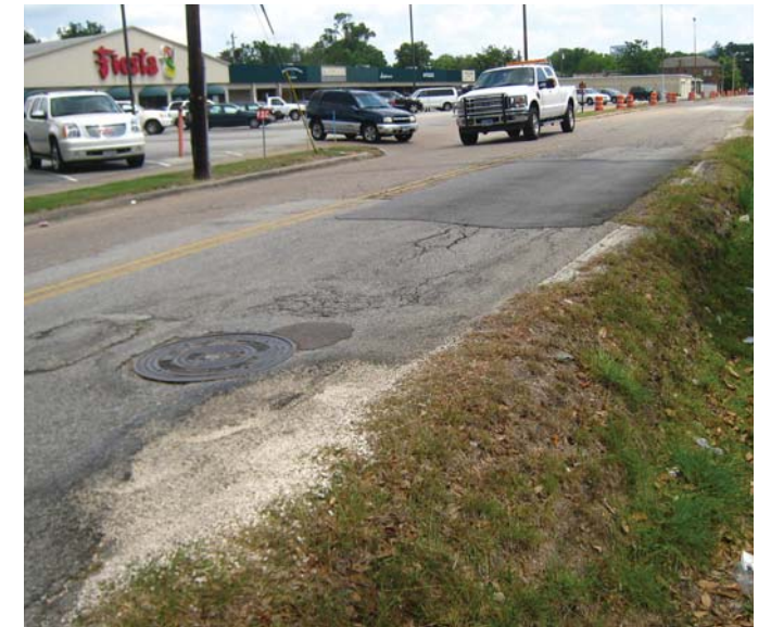
Photo 14-10, Segment 38A Dunlavy between W. Alabama and W. Main During early observations, this section of Dunlavy was uneven with some pavement missing. [This section has been rebuilt since the photo as part of a developer project.]
