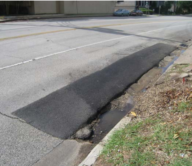
Photo 15-1, Segment 2A Shepherd between W. Dallas and McDuffie Pavement slopes off steeply near curb.
