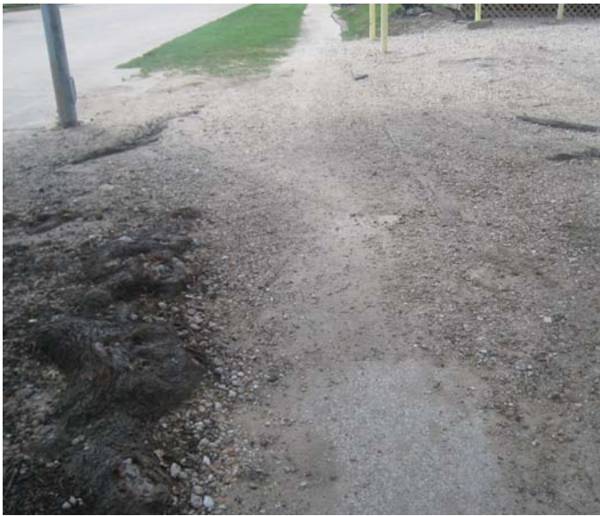
Photo 9-16, Segment 32A W. Gray between Stanford and Taft Tree roots are encroaching on the sidewalk. Dirt and pebbles accumulate on the sidewalk washed from the adjacent parking lot.
