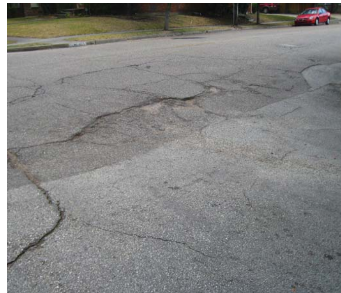
Photo 14-6, Segment 31 Dunlavy at Harold Ground settling creates uneven riding surface
