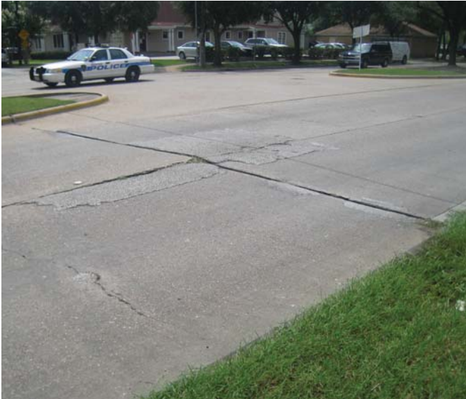
Photo 11-1, Segment 6A Montrose between W. Gray and Peden The concrete joint sealant has come out, there are cracks in the pavement, and patching is worn, creating an uneven riding surface.
