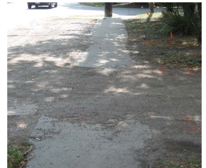
Photo 8-13, Segment 10B Fairview between Hazard and Driscoll Missing section of sidewalk
