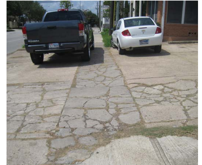
Photo 12-9, Segment 4B Waugh between W. Clay and Bell Sidewalk is severely cracked and used for the parking, making it hard to access as a pedestrian.
