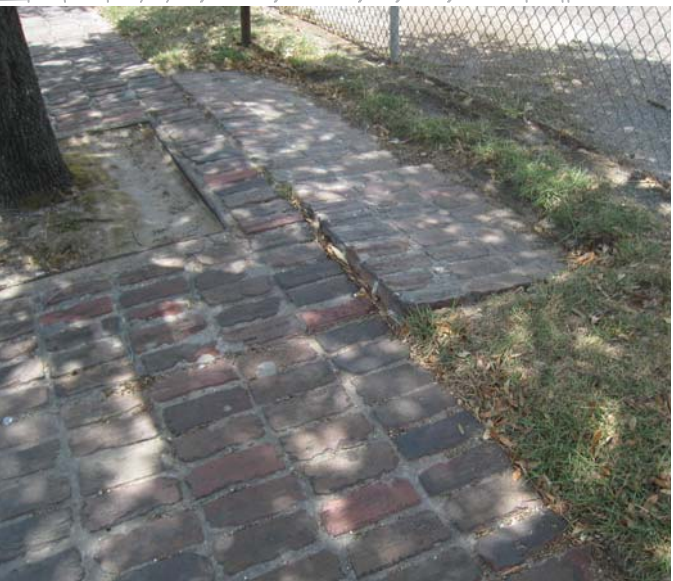
Photo 5-13, Segment 14A Between Mandell and Loretto Pavers are uneven and create tripping hazards. Passage widths are too narrow.
