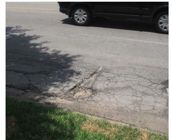
Photo 9-3, Segment 10B W. Gray between Woodhead and Dunlavy Cracking near the curb has begun to create section that have been kicked up and create potholes.
