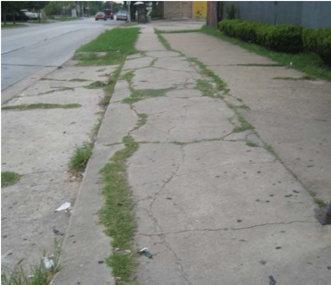
Photo 7-21, Segment 62A Westheimer between Taft and Mason Cracks in the sidewalk and grass growth in the cracks
