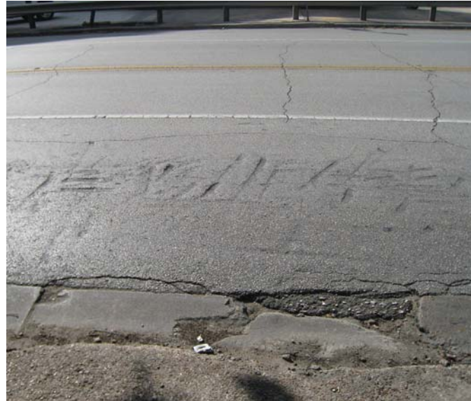
Photo 15-2, Segment 4A Shepherd between McDuffie and Newhouse Cracking and scrapes in lane
