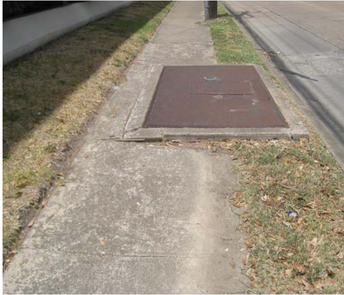
Photo 10-15, Segment 12A W. Dallas between Rosine and Waugh Sidewalk has settled around the metal utility grate, creating a tripping hazard.
