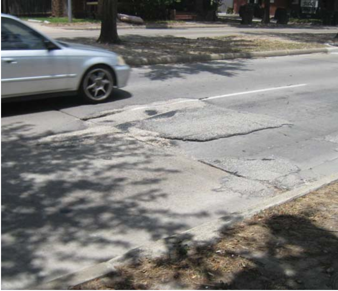
Photo 5-4, Segment 12B Richmond between Dunlavy and Mandell This section of the road appears to have been previously patched, but the patch is no longer flush with the road and there are sections missing.
