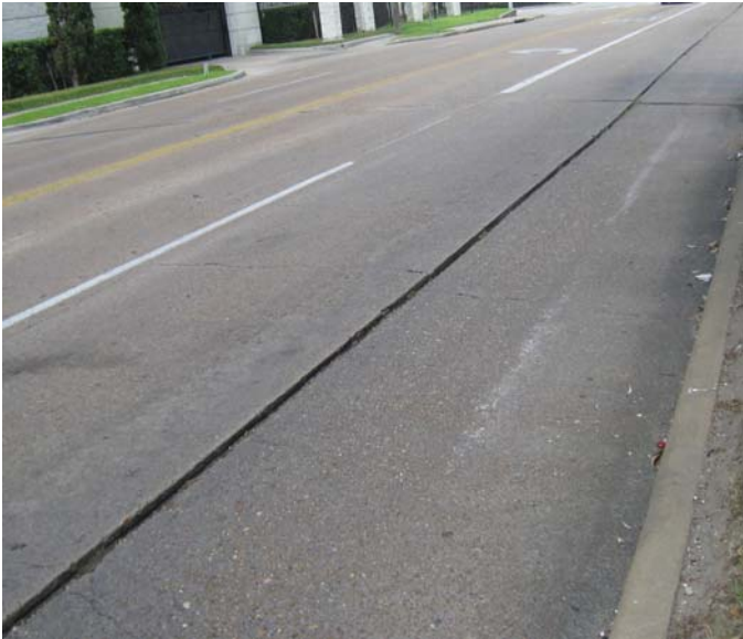
Photo 10-1, Segment 2A W. Dallas between Shepherd and Gross Pavement separation at joints
