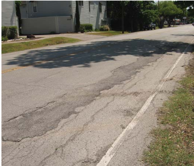
Photo 8-7, Segment 42B Fairview between Yoakum and Montrose Roadway settling that has been previously patched is uneven with remaining roadway.
