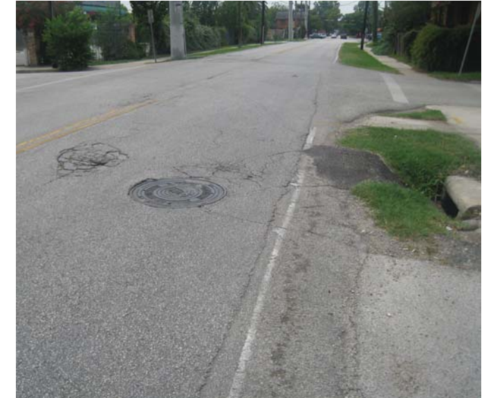
Photo 8-8, Segment 48A Fairview between Converse and Crocker Several cracks and a pothole have formed in this section of the pavement.
