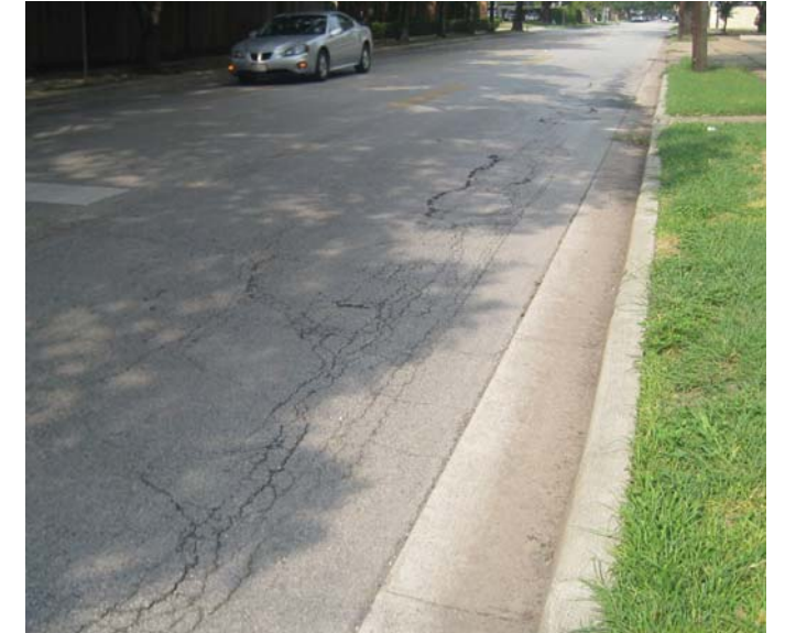
Photo 6-11, Segment 30A W. Alabama between Roseland and Stanford The cracking creates an uneven riding surface and may widen or propagate creating additional problems.
