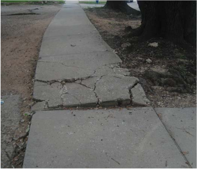
Photo 9-17, Segment 32B W. Gray between Stanford and Taft Sidewalk section is cracked by tree roots
