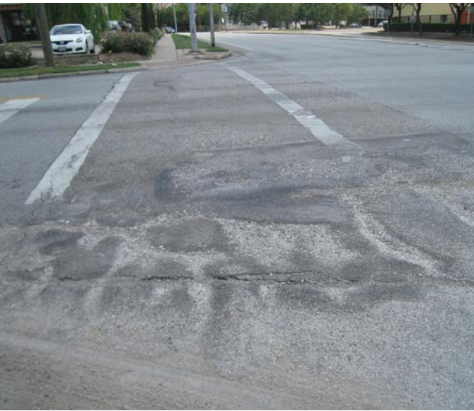
Photo 12-3, Segment 9 Waugh at W. Gray Wear pattern and settling has created an uneven surface.
