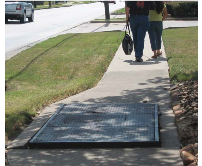
Photo 9-10, Segment 14A W. Gray between Metropolitan and Waugh Metal utility feature is not even with the sidewalk and creates a tripping hazard.
