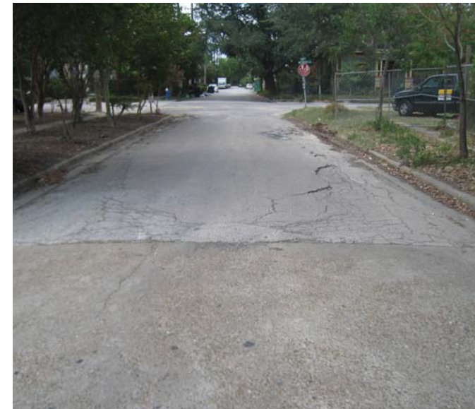
Photo 12-7, Segment 39 Waugh at Yoakum Roadway is settling unevenly near the curb.
