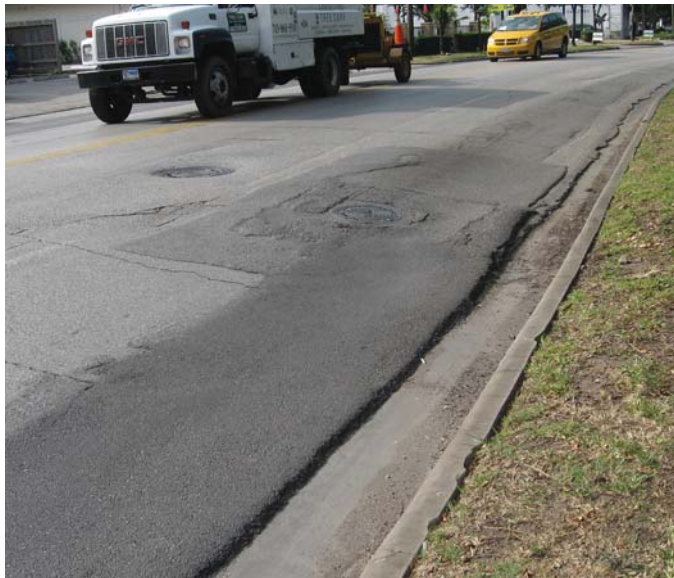
Photo 15-7, Segment 28A Shepherd between Fairview and Westheimer Patching creates drop off at curb and gutter effectively narrowing the lane.
