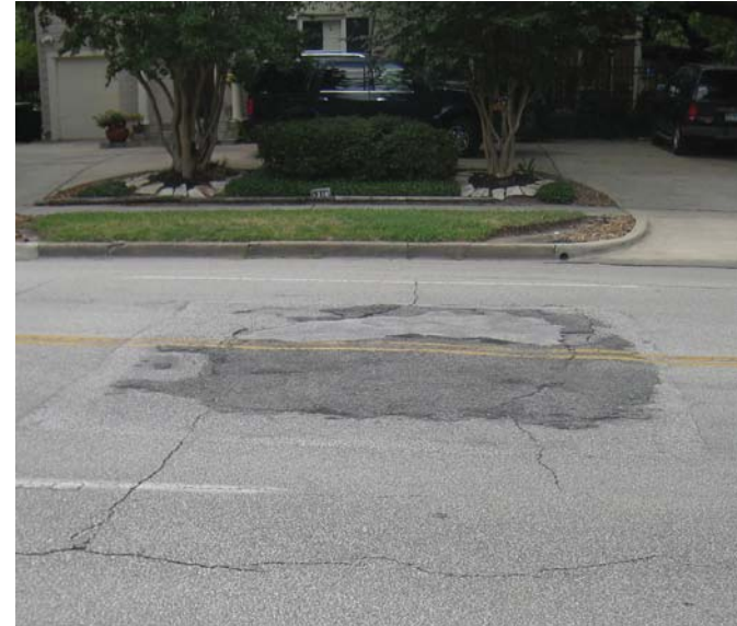
Photo 15-3, Segment 6B Shepherd between Newhouse and Pine Valley Uneven patched pavement in middle of the road
