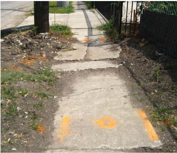
Photo 14-21, Segment 38A Dunlavy between W. Alabama and W. Main Cracking and settling
