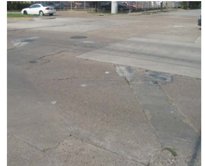
Photo 11-2, Segment 13 Montrose at Welch Numerous cracks and patching at the intersection create an uneven riding surface.
