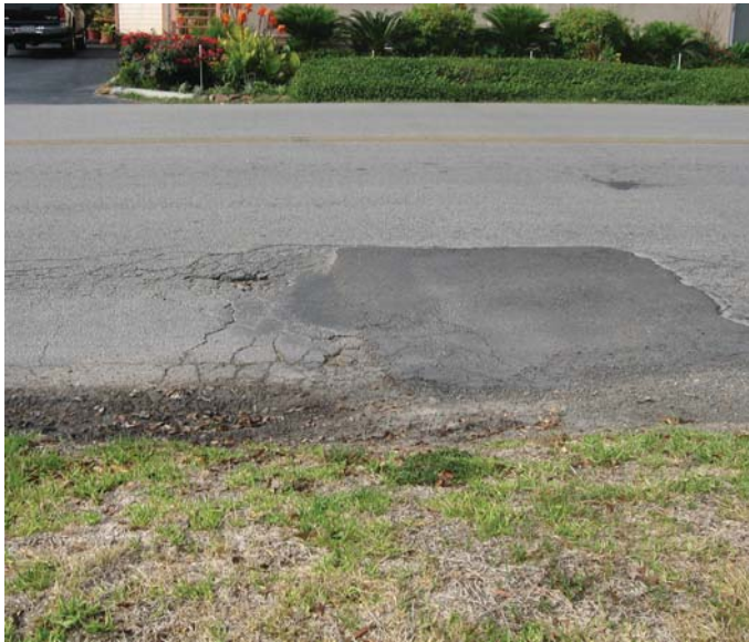
Photo 8-1, Segment 2A Fairview between Shepherd and Huld Patched pavement with cracks and missing sections just before Shepherd.
