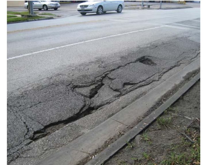
Photo 15-5, Segment 20A Shepherd between Haddon and San Felipe/Vermont Severe cracking near curb
