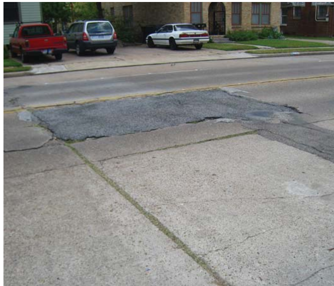
Photo 14-3, Segment 12B Dunlavy between Haddon and Vermont Previous patch shows extreme wear and is uneven.
