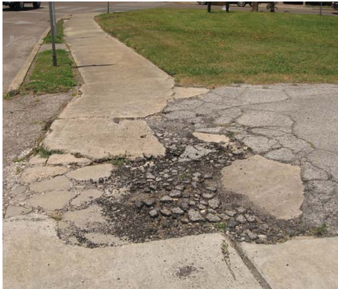
Photo 8-16, Segment 22A Fairview between Dunlavy and Ralph Broken and missing section of sidewalk creates a section that is challenging to traverse.
