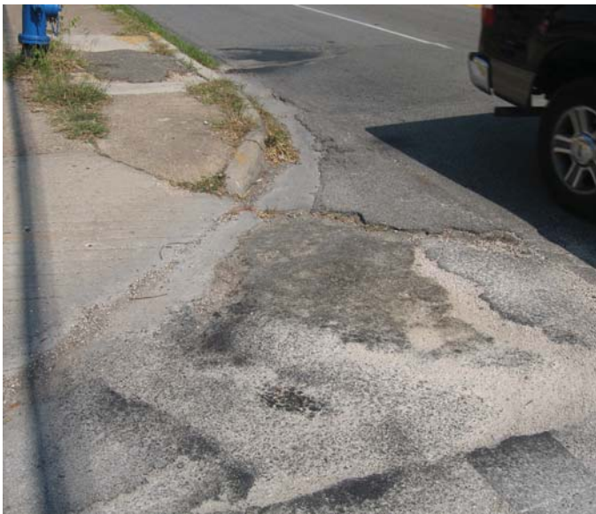
Photo 7-5, Segment 46A Westheimer between Waughcrest and Waugh Missing layer of pavement at corner
