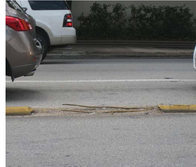
Photo 15-4, Segment 12A and 12B Shepherd between Brentwood and W. Gray/Inwood Section of the median missing and exposed rebar
