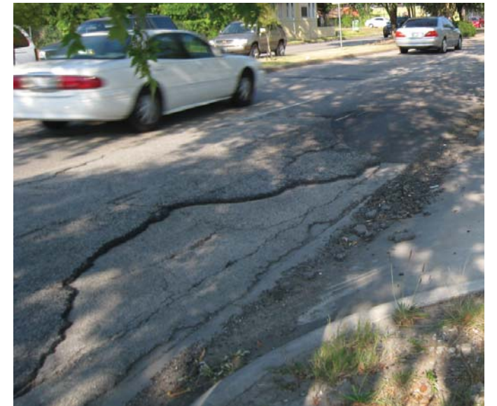
Photo 5-8, Segment 36A WB Richmond near Milam Asphalt surface overlay is worn and needs repair/ replacement.
