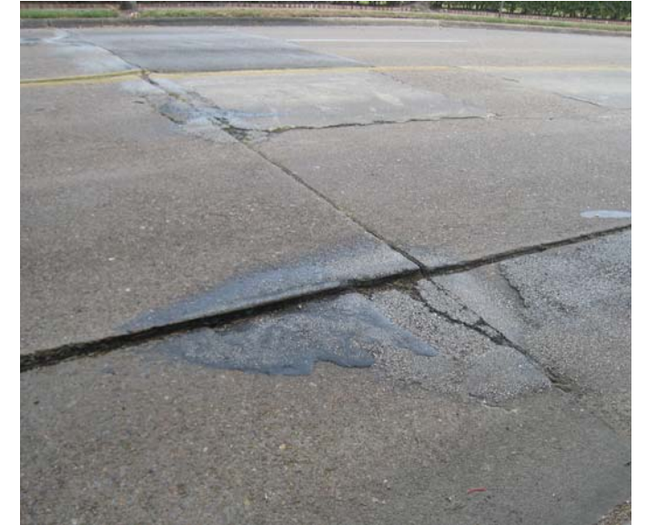
Photo 10-2, Segment 6B W. Dallas between Tirell and Dunlavy Settling creating an uneven surface
