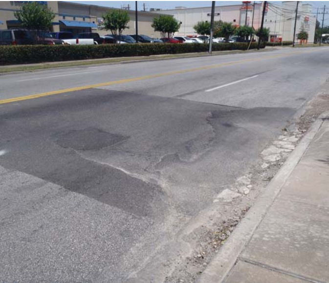
Photo 7-1, Segment 4B Westheimer between Huldy and Brun Patched pavement has settled close to the curb and created an uneven riding surface.
