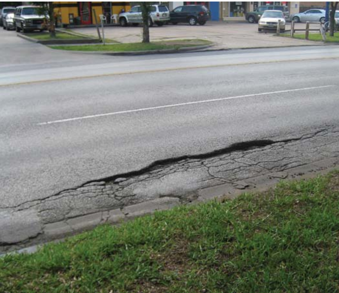
Photo 15-6, Segment 22A Shepherd between San Felipe/Vermont and Welch Severe cracking near curb
