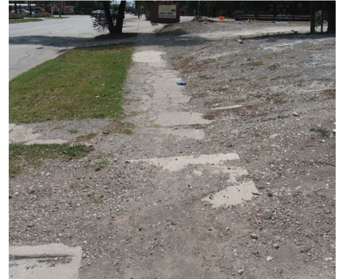
Photo 9-11, Segment 16A W. Gray between Waugh and Hazel Major portions of the sidewalk are either missing or covered by dirt and gravel.
