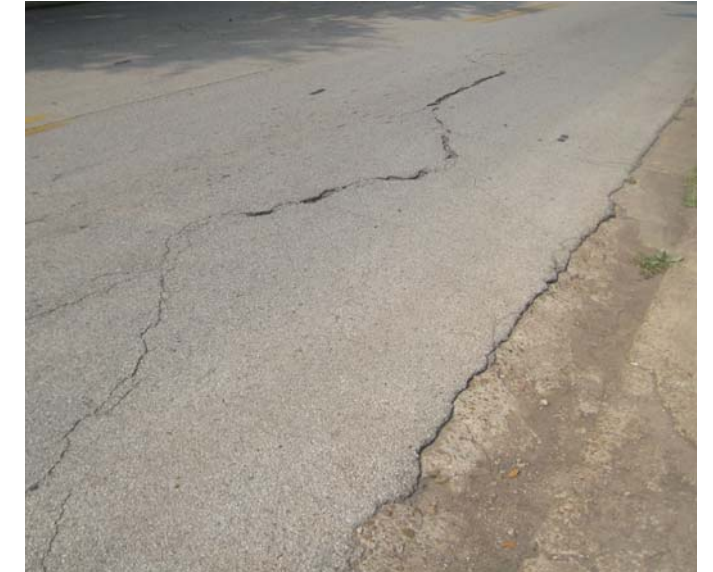
Photo 6-12, Segment 30A W. Alabama between Roseland and Stanford The cracking creates an uneven riding surface and may widen or propagate creating additional problems.
