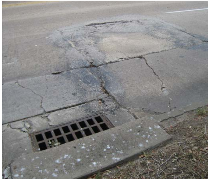
Photo 10-4, Segment 8B W. Dallas between Dunlavy and Rowchow Pavement is cracked and uneven near storm drain.
