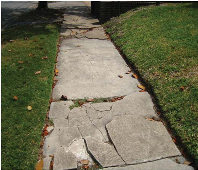
Photo 14-19, Segment 34A Dunlavy between Kipling and Marshall Cracking and settling
