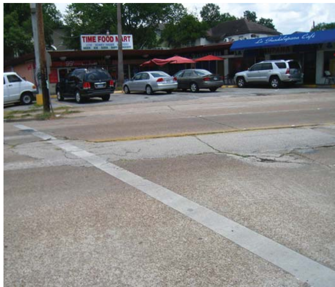
Photo 14-4, Segment 17 Dunlavy at Indiana Previous patch is cracking at the edges
