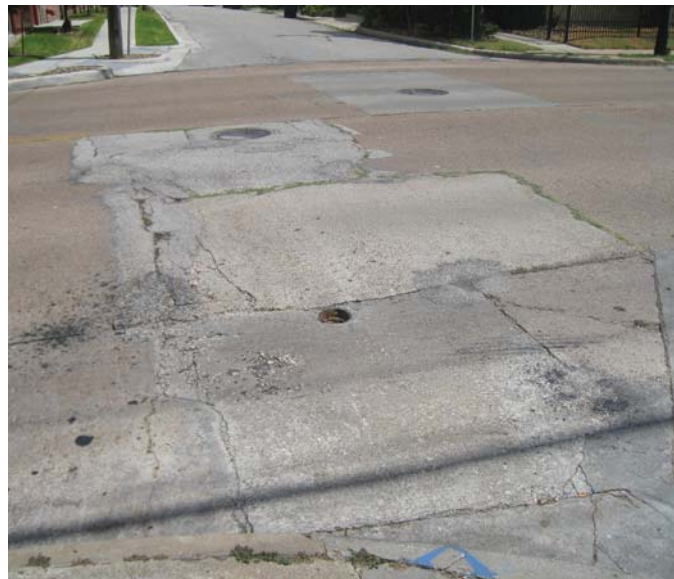
Photo 10-5, Segment 12B W. Dallas between Rosine and Waugh Several previous patches have resulted in an uneven surface.
