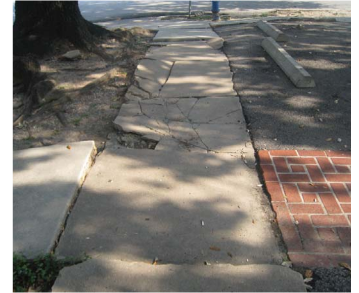
Photo 11-10, Segment 36B Montrose between Kipling and Marshall Sidewalk has severe cracking and upheaval, creating a tripping hazard.
