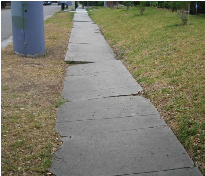
Photo 14-18, Segment 32A Dunlavy between Harold and Kipling Sidewalk sections have cracked and shifted, creating tripping hazards at the joint and cracks.
