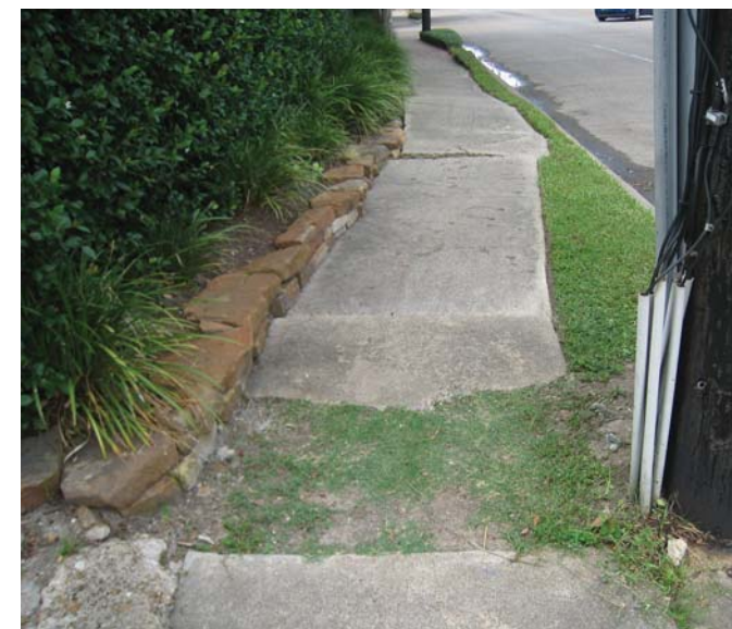
Photo 14-15, Segment 12B Dunlavy between Haddon and Vermont Missing section of sidewalk
