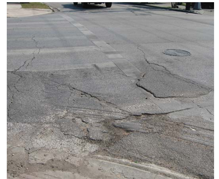
Photo 7-3, Segment 9 Westheimer at Hazard Pavement at the corner is cracked and uneven.
