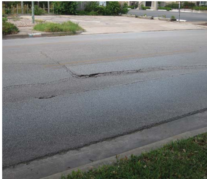
Photo 6-7, Segment 16B W. Alabama between Mandell and Mulberry The pavement has settled unevenly, creating a small drop off or fault in the center of the lane.
