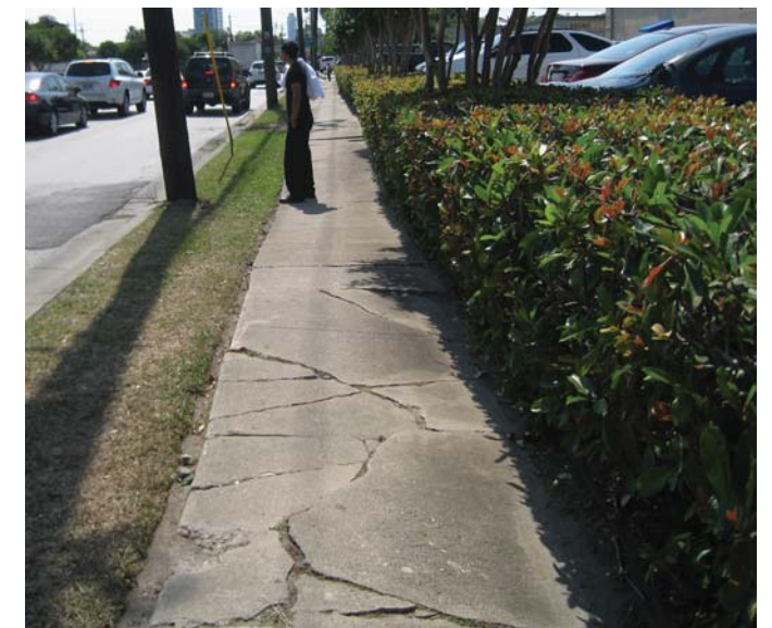
Photo 7-12, Segment 4A Westheimer between Huldy and Brun Sidewalk is cracked and has settled, creating tripping hazards.
