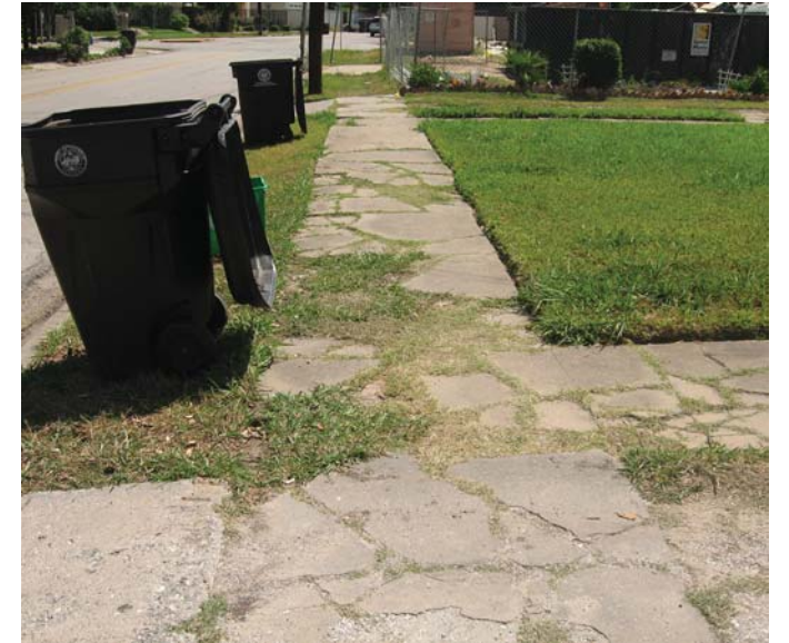
Photo 8-21, Segment 32B Fairview between Yupon and Commonwealth Sidewalk is cracked and sections are missing.
