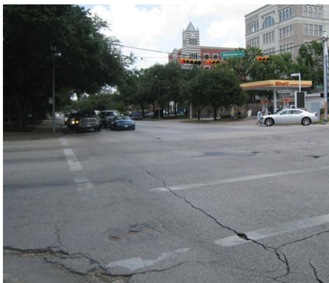
Photo 5-7, Segment 25 Richmond at Montrose Cracks, potholes, and patching creates an uneven riding surface.
