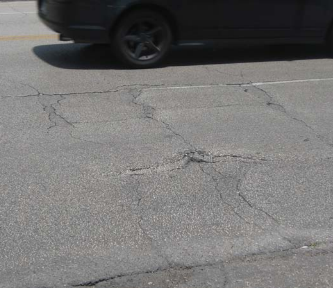
Photo 9-1, Segment 4B W. Gray between Driveway and McDuffie Pavement settling has created an uneven riding surface.
