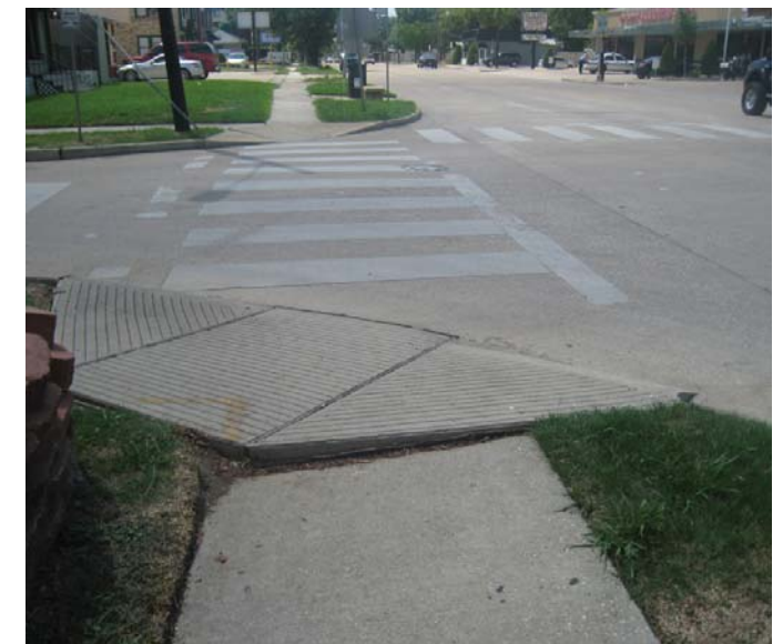
Photo 9-15, Segment 31 W. Gray at Stanford Settling has separated the sidewalk from the ramp on the southeast corner.
