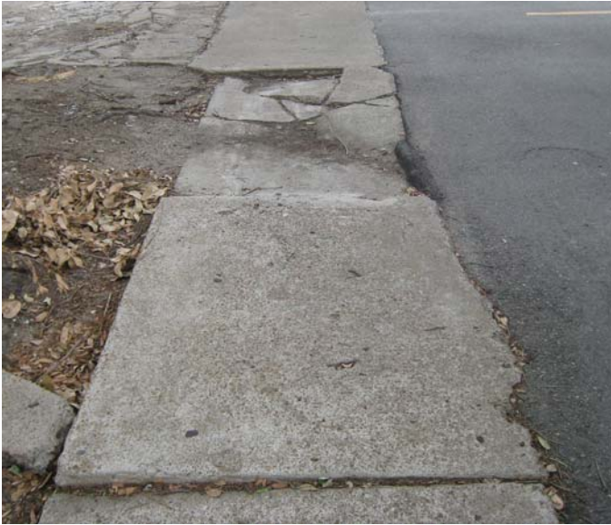
Photo 13-12, Segment 18A Commonwealth between Hyde Park and Missouri Sidewalk settling and cracking
