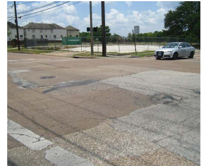
Photo 14-1, Segment 1 Dunlavy at W. Dallas Patching creates an uneven riding surface
