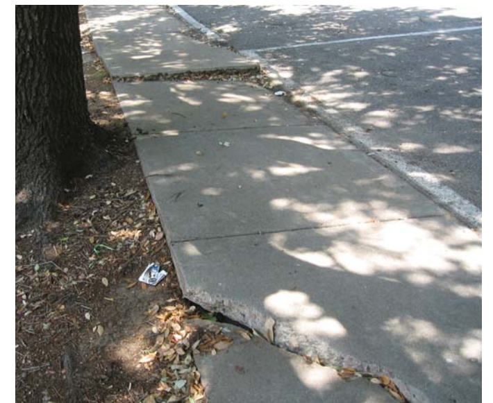
Photo 6-19, Segment 18A W. Alabama between Mulberry and Yupon Sections have broken off, creating tripping hazards.
