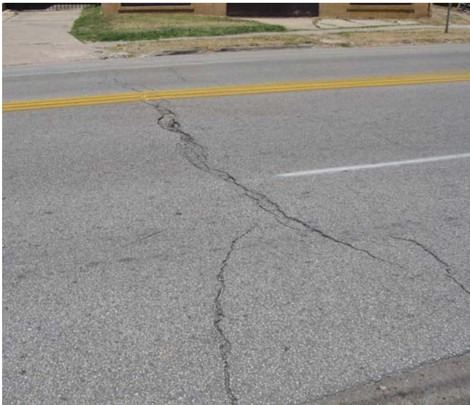
Photo 7-4, Segment 40B Westheimer between Graustark and Commonwealth Large crack across the width of the lanes
