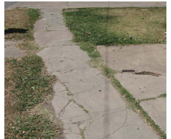
Photo 7-18, Segment 38A Westheimer between Yupon and Graustark Sidewalk is broken and edges are starting to settle away from the main walkway.
