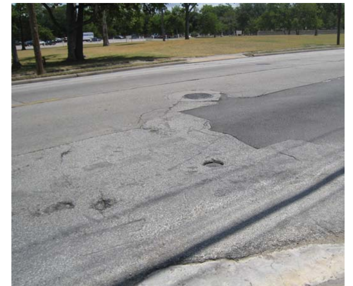
Photo 10-8, Segment 27 W. Dallas at Marconi Potholes at locations where utility connections have not been adjusted after an overlay.
