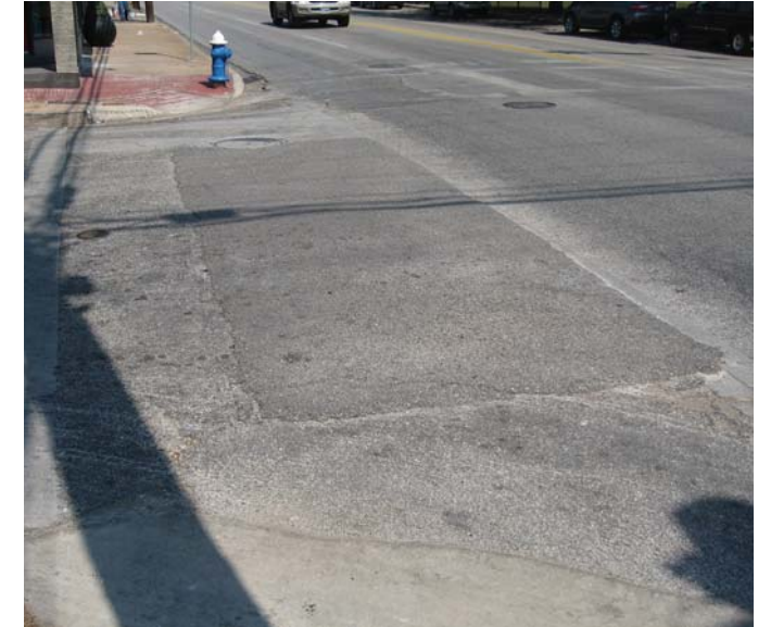
Photo 7-6, Segment 49 Westheimer at Lincoln Pavement patch uneven with the original surface
