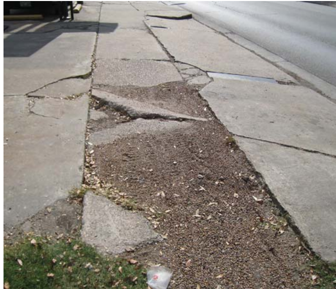
Photo 6-20, Segment 18B W. Alabama between Mulberry and Yupon Sidewalk is cracked, missing, and covered in dirt, making it difficult to traverse.
