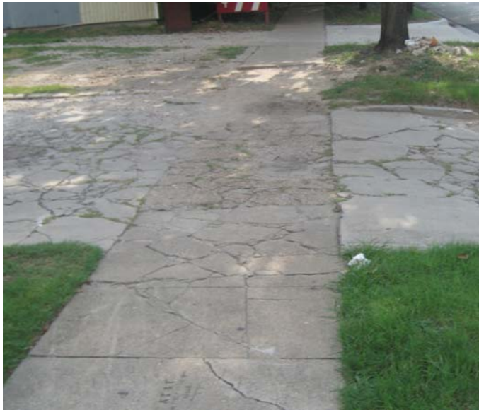
Photo 6-25, Segment 38A W. Alabama between Audubon and Garrott There is substantial cracking.
