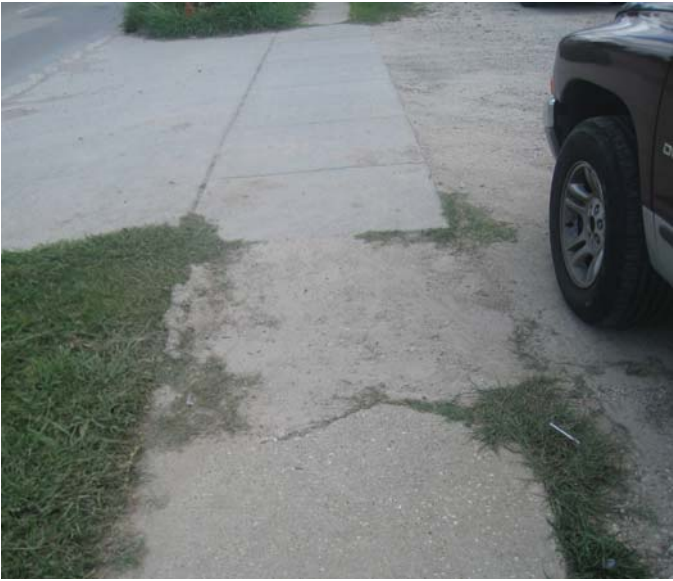
Photo 9-18, Segment 32B W. Gray between Stanford and Taft Missing section of sidewalk
