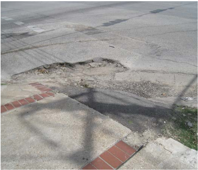
Photo 12-11, Segment 9 Waugh at W. Gray Broken ramp was patched with a steep grade. A section of pavement is missing
