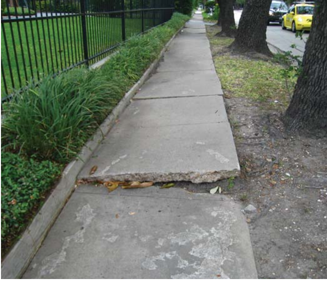
Photo 14-20, Segment 36A Dunlavy between W. Main and Colquitt Tree root has caused sidewalk to break and lift
