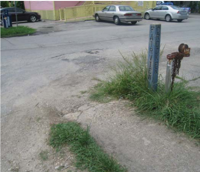
Photo 8-24, Segment 49 Fairview at Crocker Missing intersection ramps
