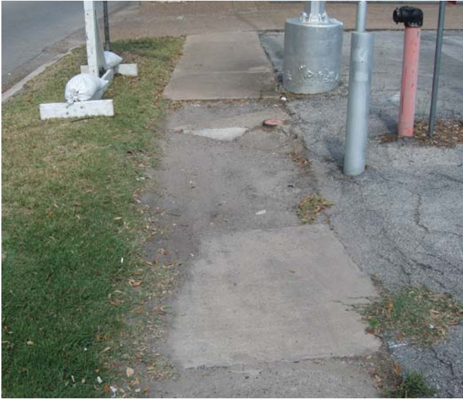
Photo 6-17, Segment 14B W. Alabama between Dunlavy and Mandell Untrimmed vegetation and missing section.
