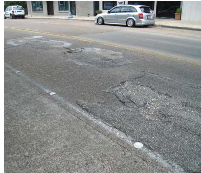
Photo 14-5, Segment 22A Dunlavy between Maryland and Fairview Uneven pavement and pot holes, with evidence of possible patching.
