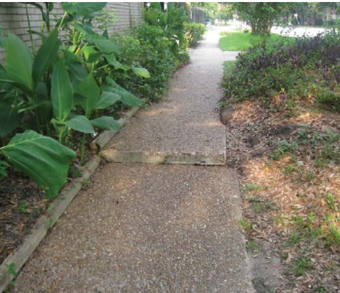
Photo 6-24, Segment 40B W. Alabama Between Garrott and Bute There is substantial upheaval at the sidewalk joint.
