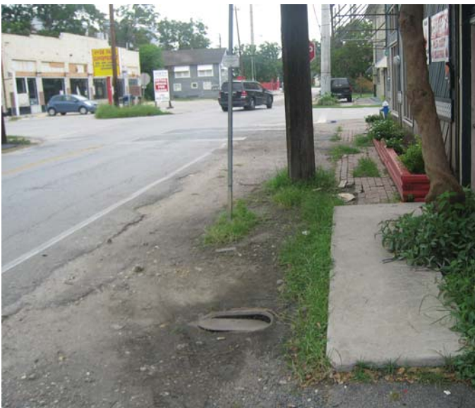
Photo 8-26, Segment 58B Fairview between Morgan and Taft Narrow and uneven sidewalk with inconsistent use of materials
