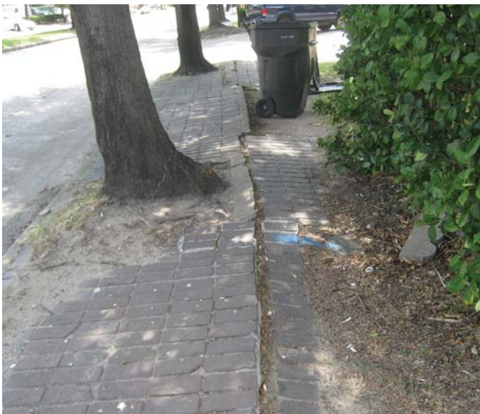
Photo 5-11, Segment 8A Between Driscoll and Woodhead Pavers are uneven and create tripping hazards.
