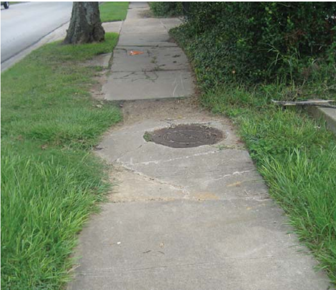
Photo 6-23, Segment 28B W. Alabama between Montrose and Roseland Portions of the sidewalk have cracks and upheaval, and some portion is missing.
