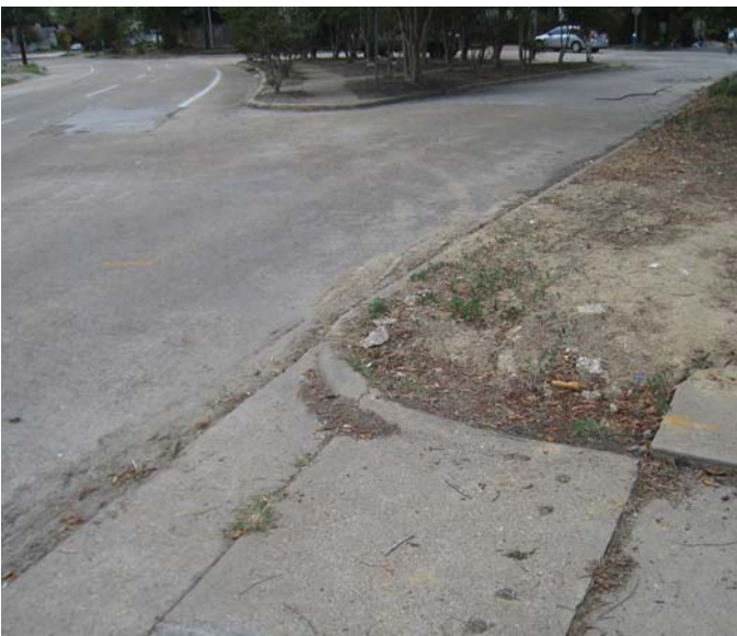
Photo 12-19, Segment 39 Waugh at Yoakum Missing ramps
