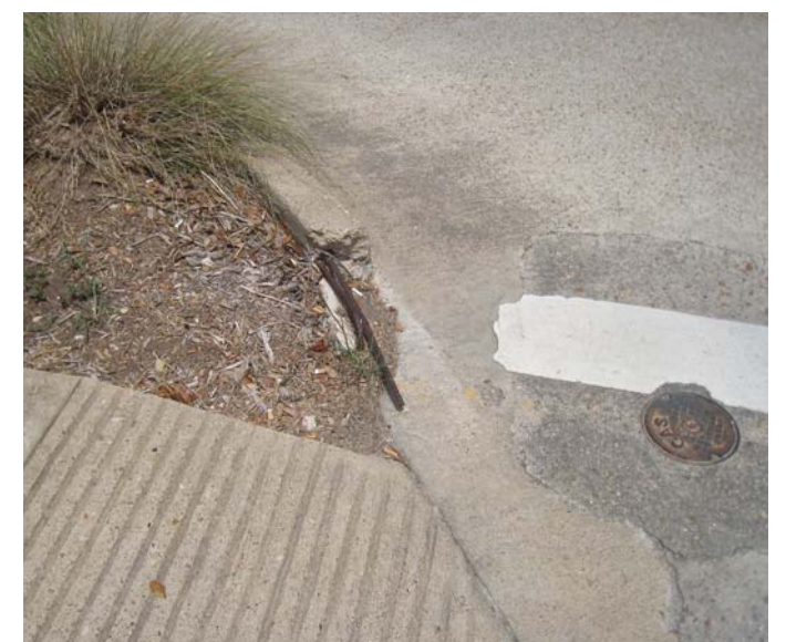
Photo 12-10, Segment 7 Waugh at Pierce Curb is broken at the ramp, exposing rebar.
