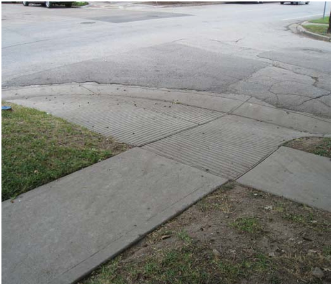
Photo 13-13, Segment 21 Commonwealth at California Ramp appears to be non-compliant to ADA standards
