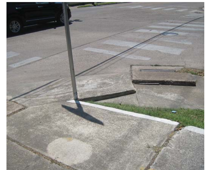
Photo 8-15, Segment 21 Fairview at Dunlavy Settling of the sidewalk at the ramp and drain has created a tripping hazard.
