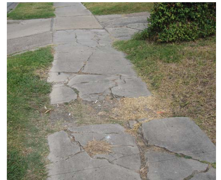
Photo 6-16, Segment 12B W. Alabama between Woodhead and Dunlavy Missing sections, cracking, and uneven settling create tripping hazards.
