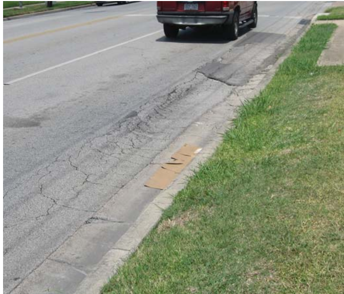
Photo 9-5, Segment 12B W. Gray between Dunlavy and Metropolitan Settlement has created alligator cracking.
