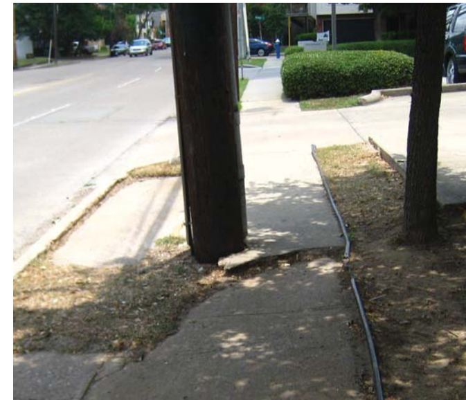
Photo 14-14, Segment 8B Dunlavy between W. Gray and Peden Settling and obstructions
