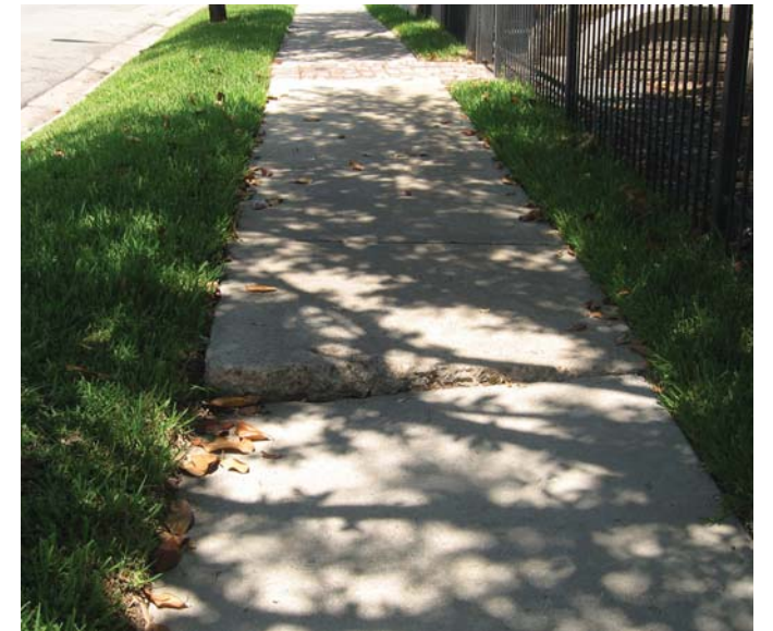
Photo 8-14, Segment 14A Fairview between Morse and Woodhead Sidewalk upheaval has created a tripping hazard.
