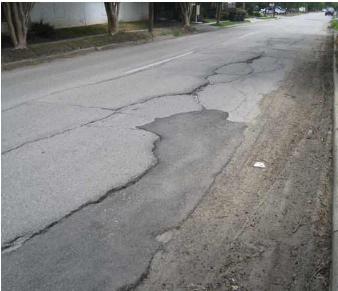
Photo 12-4, Segment 16A Waugh between Vermont and Welch Prior patching and further settlement have created an uneven surface.
