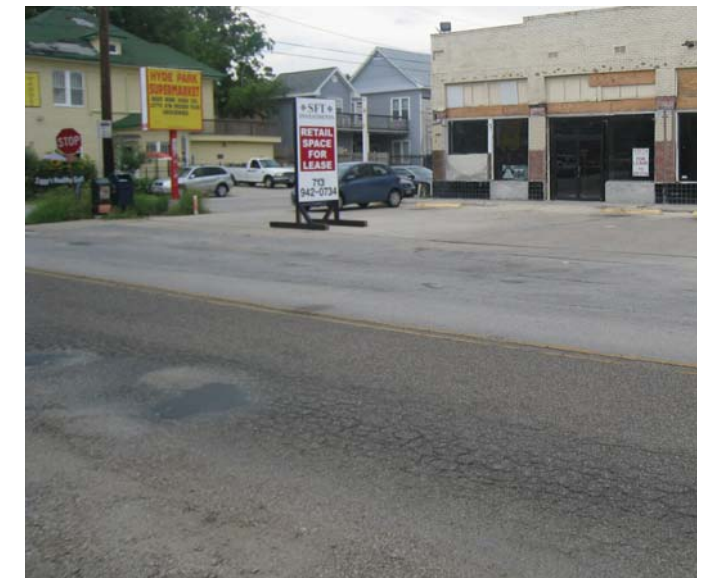
Photo 8-9, Segments 60A & 60B Fairview between Taft and Mason Eastbound lanes are weathered forming cracks. Westbound section has multiple potholes.
