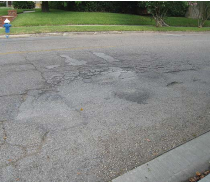
Photo 14-9, Segment 34B Dunlavy between Kipling and Marshall Alligator cracking and uneven settling, with evidence of previous patches
