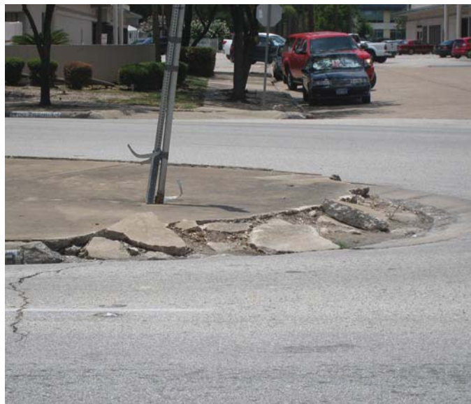
Photo 15-8, Segment 49 Shepherd at Portsmouth Median is cracked and broken. Chunks are displaced, creating possible traffic hazards.
