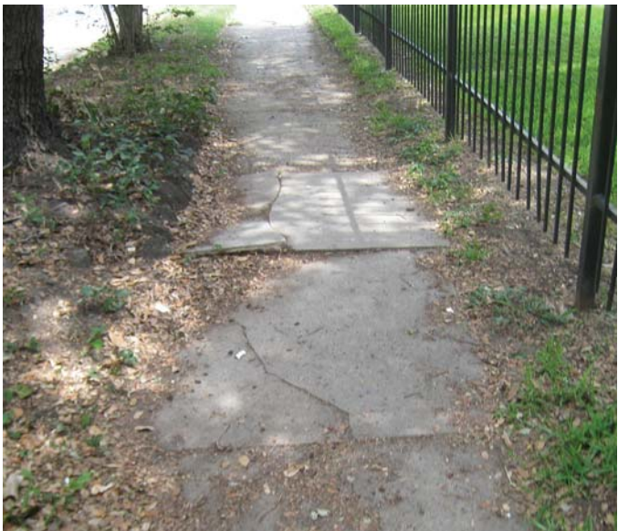
Photo 12-17, Segment 32A Waugh between Hyde Park and Missouri Roots have caused sidewalk movement and tripping hazards.
