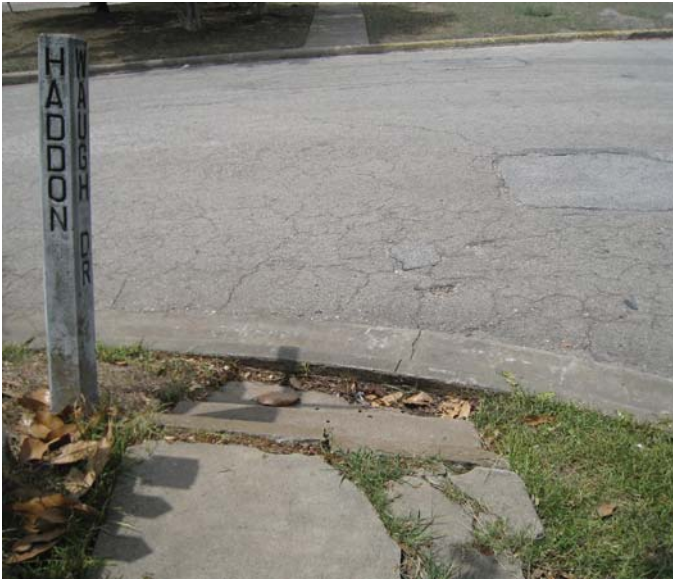
Photo 12-12, Segment 11 Waugh at Haddon/Peden Ramp missing
