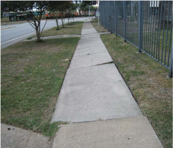
Photo 12-14, Segment 14B Waugh between Nevada and Vermont Whole sidewalk is on an angle
