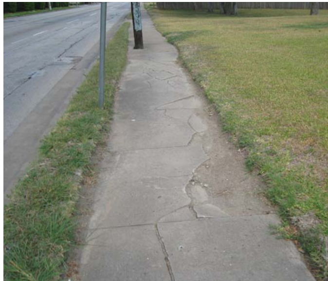
Photo 10-16, Segment 24A W. Dallas between Van Buren and Wilkenson Sidewalk is cracked, and sections are missing near the edge.
