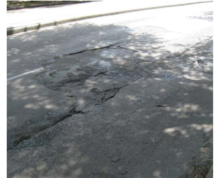
Photo 5-2, Segment 4A Richmond between McDuffie and Hazard Shows a close up of the cracks and general deterioration which create an uneven riding surface
