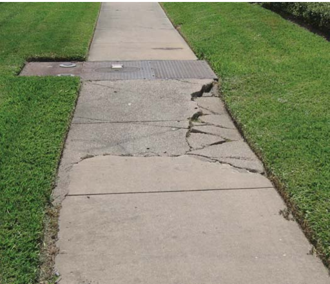
Photo 9-9, Segment 12A W. Gray between Dunlavy and Metropolitan Cracking of the sidewalk
