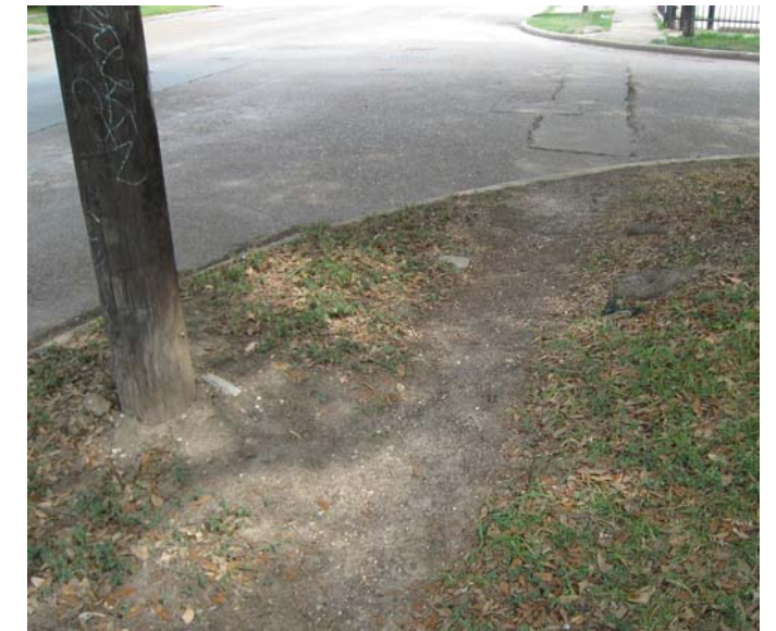
Photo 13-7, Segment 3 Commonwealth at Nevada Missing sidewalk and ramp
