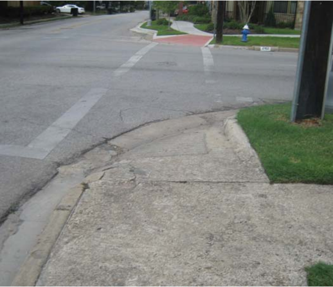
Photo 13-11, Segment 15 Commonwealth at Fairview Appears to be a non-compliant ramp (too steep and too short)
