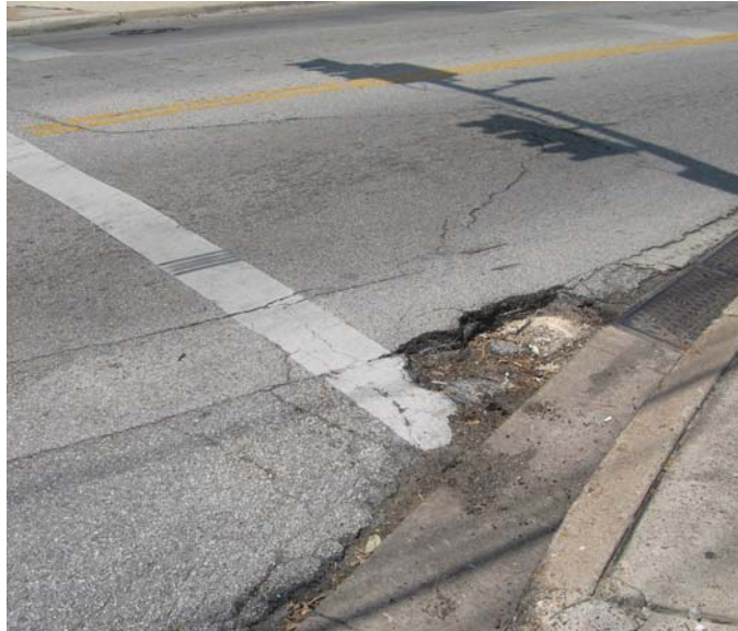
Photo 6-1, Segment 2B W. Alabama between Shepherd and Huldy A section of the asphalt is missing near the Shepherd intersection.
