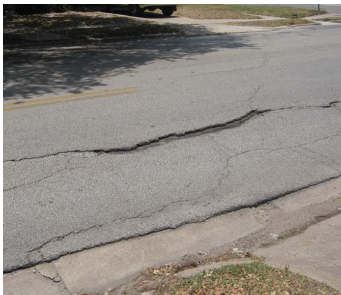
Photo 6-8, Segment 20A W. Alabama between Yupon and Graustark The pavement has settled unevenly, creating a small drop off or fault in the center of the lane.
