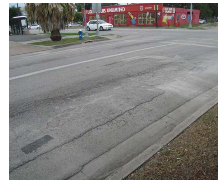
Photo 13-5, Segment 22A Commonwealth between California and Westheimer Alligator cracking near intersection
