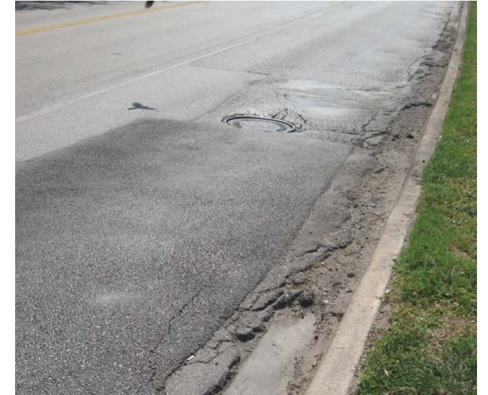
Photo 7-2, Segment 6A Westheimer between Brun and McDuffie Pavement around the patch is crumbling and coming up, additionally the roadway is uneven and has visible ruts where tires traditionally travel.
