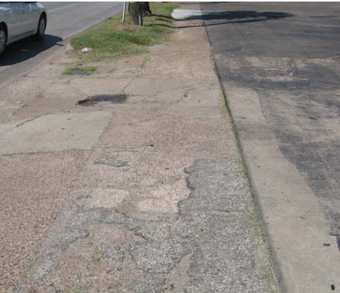
Photo 7-19, Segment 44A Westheimer between Mt. Vernon and Waughcrest Excess asphalt on top of existing sidewalk creates tripping hazards.
