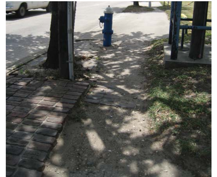
Photo 5-17, Segment 20A Richmond between Graustark and Mt. Vernon Missing pavers create uneven surface. Obstructions in the pedestrian path make it difficult for pedestrians to travel on the sidewalk.
