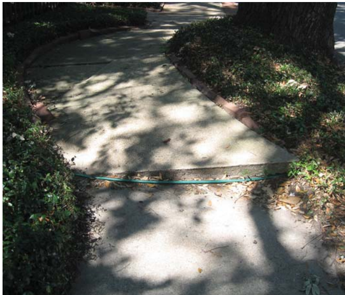
Photo 8-19, Segment 30B Fairview between Windsor and Yupon Tree root growth has shifted whole section of the sidewalk, creating a tripping hazard.
