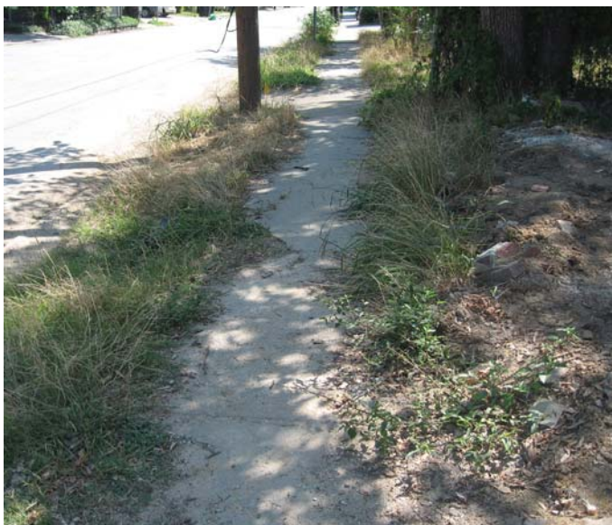
Photo 8-20, Segment 32B Fairview between Yupon and Commonwealth Sidewalk is cracked, and adjacent landscaping has started to overtake the sidewalk, narrowing the passable area.
