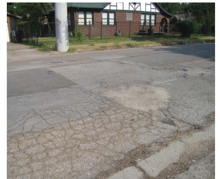
Photo 14-11, Segment 40A and 40B Dunlavy between W. Main and Colquitt Alligator cracking in travel lanes
