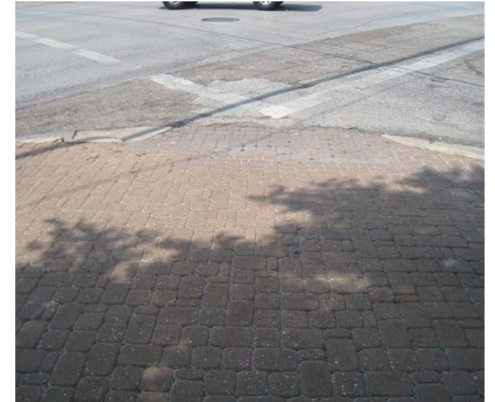
Photo 9-8, Segment 11 W. Gray at Dunlavy Non-compliant ramp
