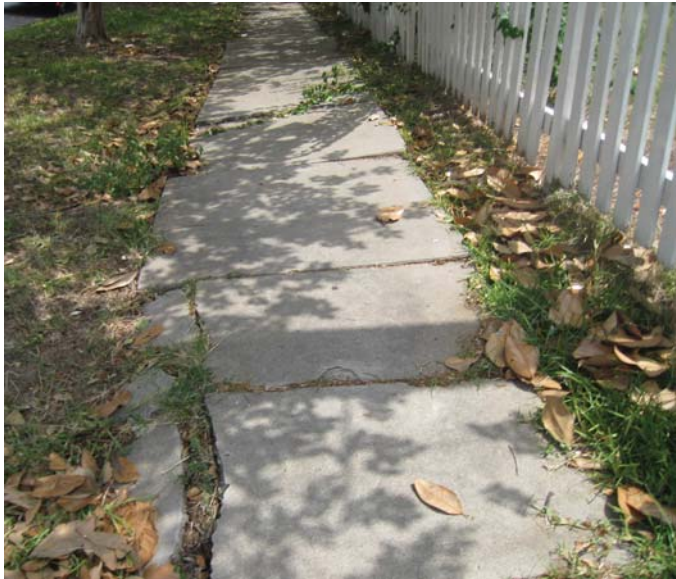
Photo 12-13, Segment 12A Waugh between Haddon/Peden and Nevada Sidewalk cracking and settling
