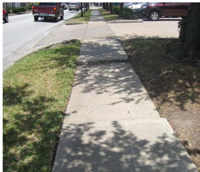
Photo 15-13, Segment 50B Shepherd between Portsmouth and Norfolk One section of sidewalk has settled, creating tripping hazards.
