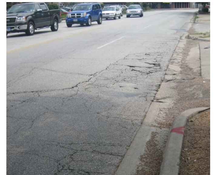
Photo 7-7, Segment 52B Westheimer between Montrose and Grant Alligator cracks along the outside lane
