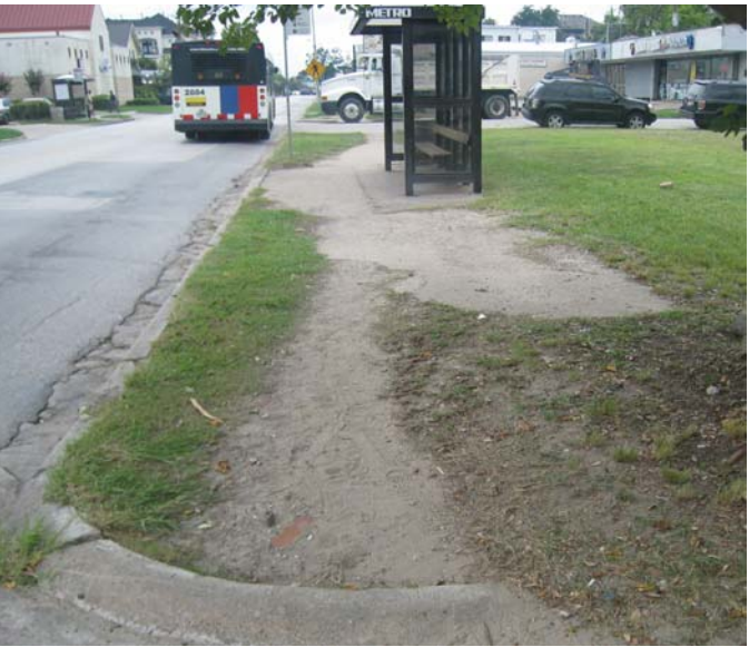
Photo 7-23, Segment 66A Westheimer between Helena and Bagby Missing section of sidewalk and ramp on the approach to bus shelter.
