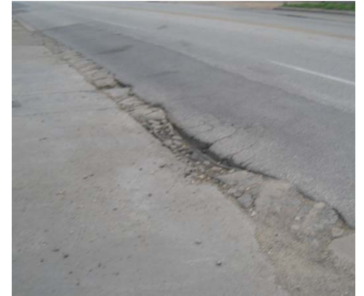
Photo 7-10, Segment 64A Westheimer between Mason and Helena Patched pavement section has cracks, and concrete in the gutter section is broken and steel is exposed.
