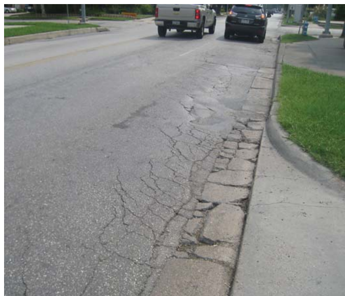
Photo 7-9, Segment 60B Westheimer between Whitney and Taft Severe cracking can be seen in the pavement and gutter sections.
