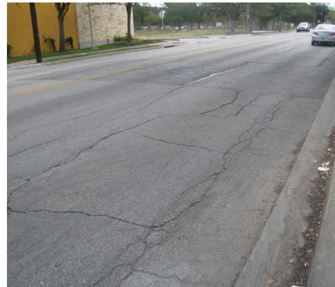
Photo 10-6, Segment 14B W. Dallas between Waugh and Peveto Long cracks create a ladder shape throughout this section of W. Dallas.
