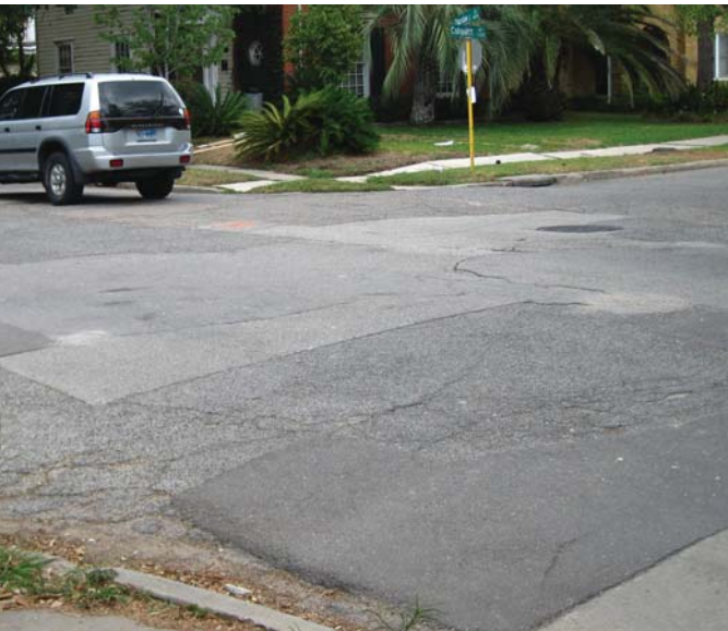
Photo 14-12, Segment 41 Dunlavy at Colquitt Cracking in the intersection and numerous previous patches
