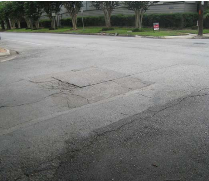
Photo 13-2, Segment 9 Commonwealth at Indiana Uneven roadway surface with small cracks.
