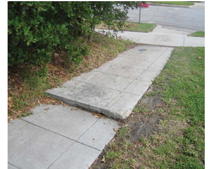
Photo 15-9, Segment 18A Shepherd between Pelham and Haddon Sidewalk section has shifted, causing tripping hazard.
