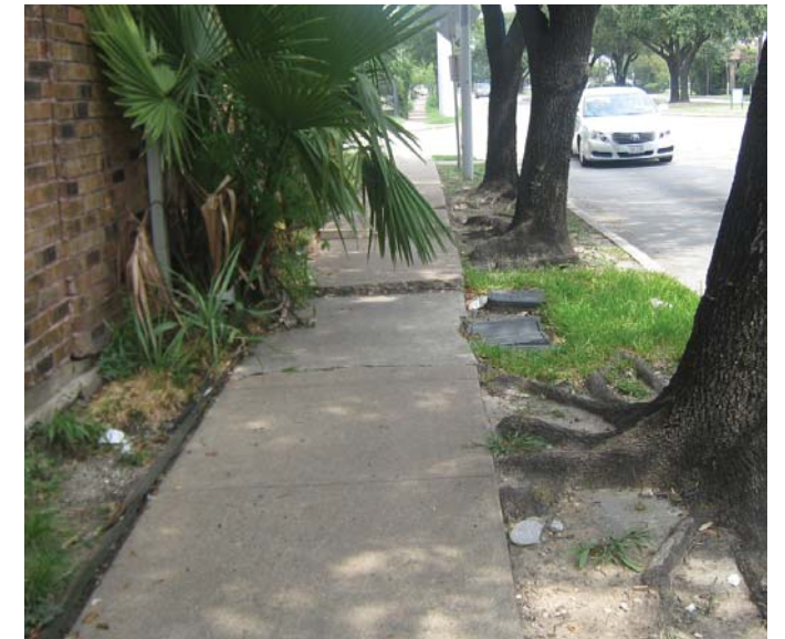
Photo 11-7, Segment 18A Montrose between Jackson and Fairview Upheaval between two sections of sidewalk and the adjacent vegetation growth obstruct pedestrian path.
