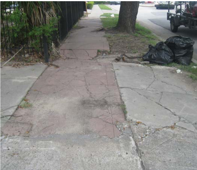
Photo 7-22, Segment 66A Westheimer between Helena and Bagby Cracks and missing section of sidewalk, with upheaval between broken sections of the sidewalk.
