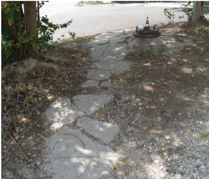
Photo 12-16, Segment 21 Waugh at W. Drew Broken sidewalk with numerous tripping hazards and no ramp
