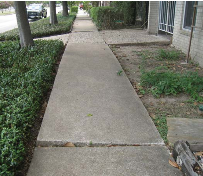
Photo 13-9, Segment 8B Commonwealth between Welch and Indiana Sidewalk section has shifted, creating both a slant and a tripping hazard.
