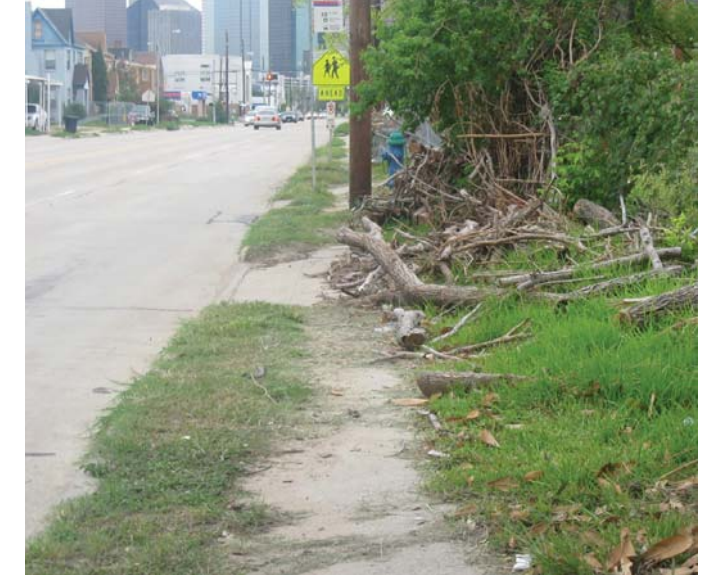
Photo 10-19, Segment 36B W. Dallas between Stanford and Taft Grass growth, debris and pole obstruction in the middle of the sidewalk
