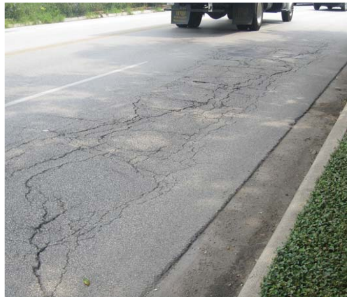
Photo 7-8, Segment 54B Westheimer between Grant and Crocker Alligator cracks along the outside lane
