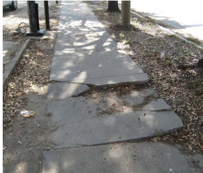
Photo 6-21, Segment 20B W. Alabama between Yupon and Graustark Broken pieces of the sidewalk create tripping hazards.
