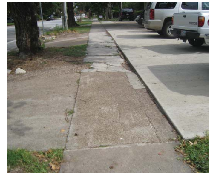
Photo 13-8, Segment 8A Commonwealth between Welch and Indiana Sidewalk has settled and is no longer flush with the adjacent pavement, creating a tripping hazard.
