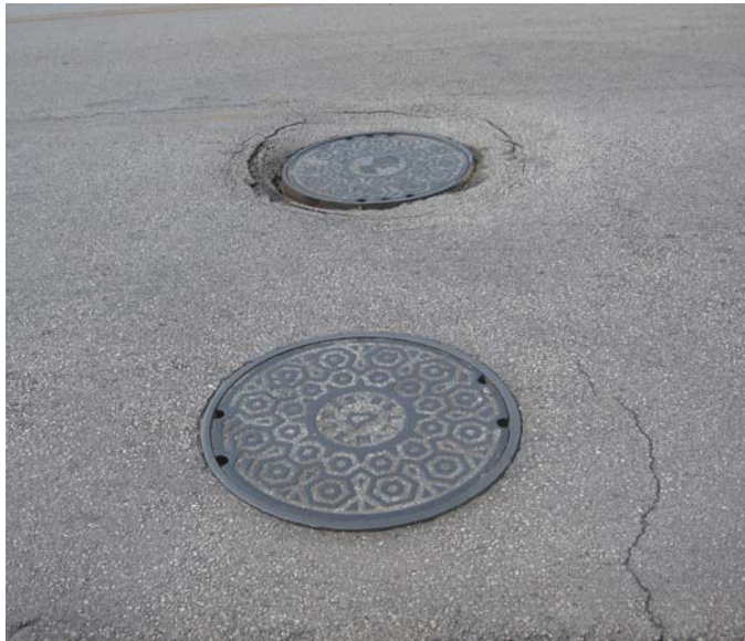
Photo 6-5, Segment 14B W. Alabama between Dunlavy and Mandell One of the manholes is significantly lower in relation to both the roadway and the other manhole.
