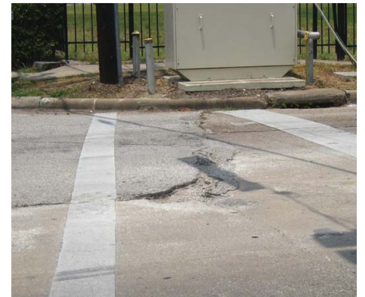
Photo 10-3, Segment 7 W. Dallas at Dunlavy Edges of a previous patch have begun to wear and have chipped away creating a noticeable bump.
