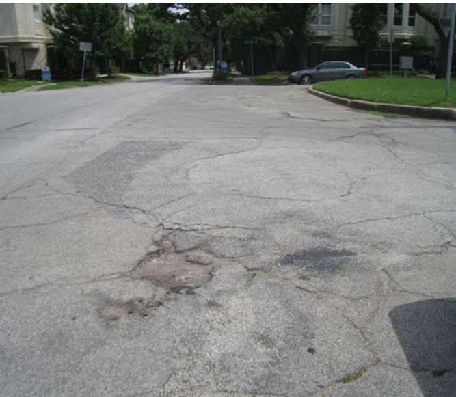
Photo 12-6, Segment 31 Waugh at Hyde Park Cracking in the intersection, with sections that are missing
