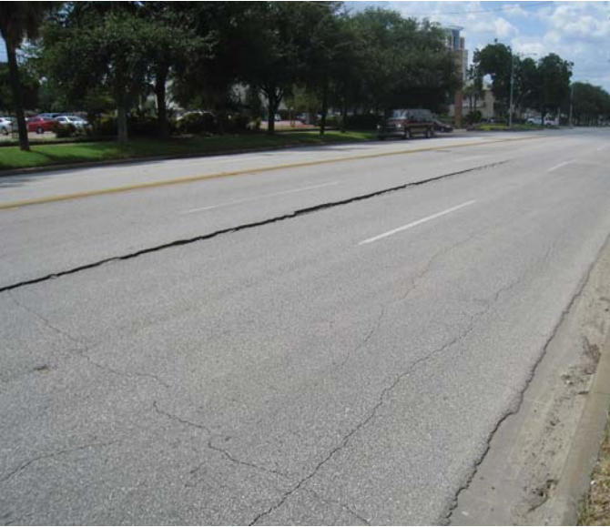
Photo 12-2, Segment 6B Waugh between Bell and Pierce Fault crack parallel to vehicular path.
