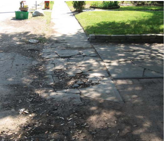
Photo 8-18, Segment 26B Fairview between Mandell and Ridgewood Sidewalk is cracked with sections missing and loose.
