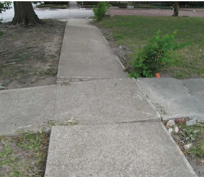
Photo 13-10, Segment 12A Commonwealth between Michigan and Maryland Path to a house has settled in comparison to the adjacent sidewalk, creating of tripping hazards.
