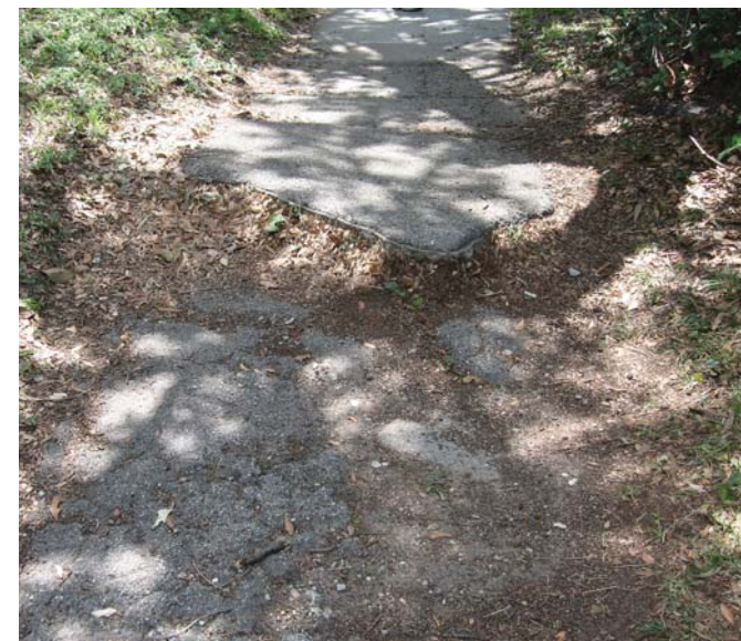
Photo 9-14, Segment 22B W. Gray between Van Buren and Marconi Uneven settling creates a tripping hazard
