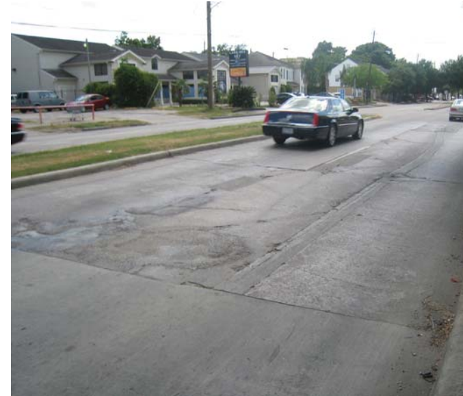
Photo 5-1, Segment 4A Richmond between McDuffie and Hazard Shows cracks and general deterioration which create an uneven riding surface
