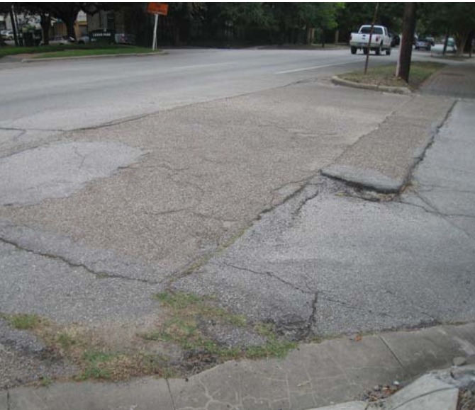
Photo 13-4, Segment 17 Commonwealth at Hyde Park One section of the pavement is raised above the rest, creating an abrupt speed bump.
