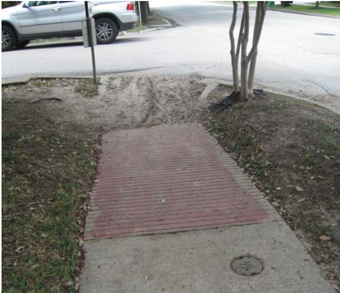
Photo 12-15, Segment 15 Waugh at Vermont End of ramp missing or covered in dirt
