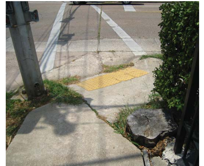
Photo 10-13, Segment 7 W. Dallas at Dunlavy Narrow sidewalk and steep ramp
