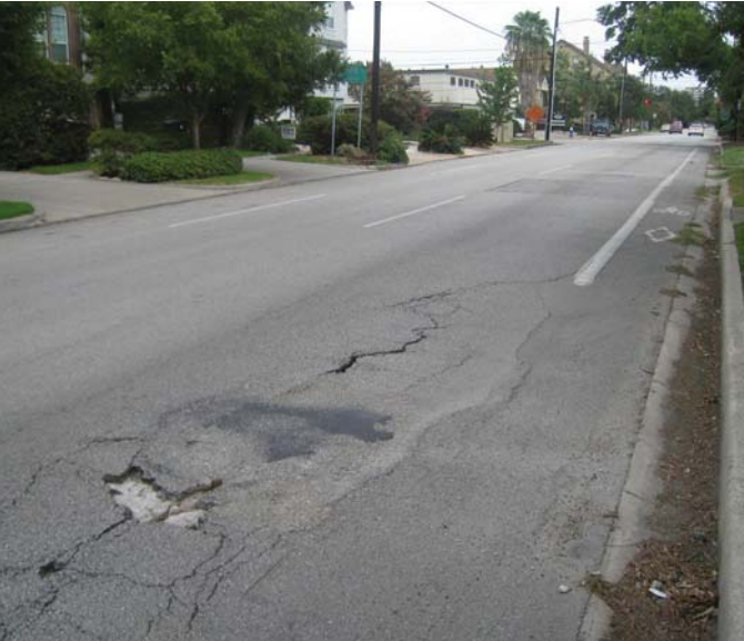
Photo 13-3, Segment 12A Commonwealth between Michigan and Maryland Cracking with small sections of pavement missing that create pot holes.
