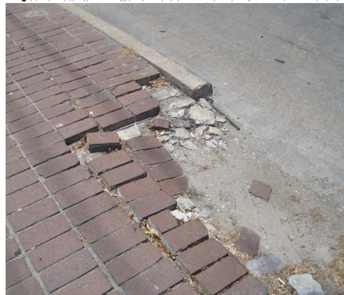
Photo 5-12, Segment 10B Between Woodhead and Dunlavy Pavers and curb are missing or broken creating a tripping hazard .
