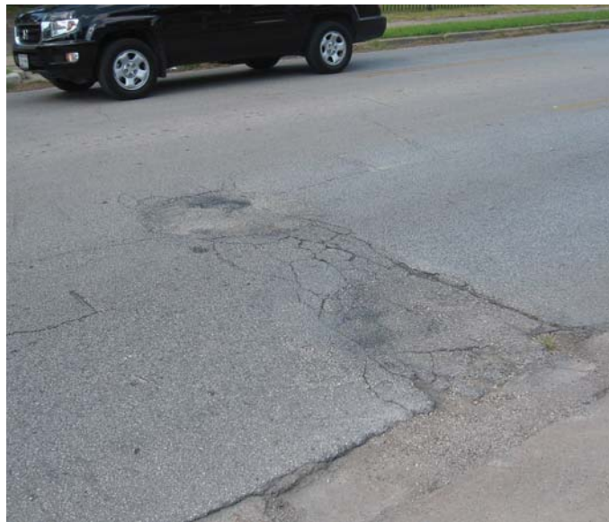
Photo 6-4, Segment 12B W. Alabama between Woodhead and Dunlavy A section of the roadway has sunken, creating a pothole.
