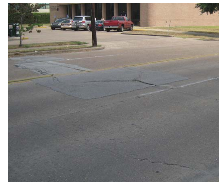
Photo 14-2, Segment 6A and 6B Dunlavy between W. Bell and W. Gray Patch is lower than the surrounding pavement, creating a depressed section.
