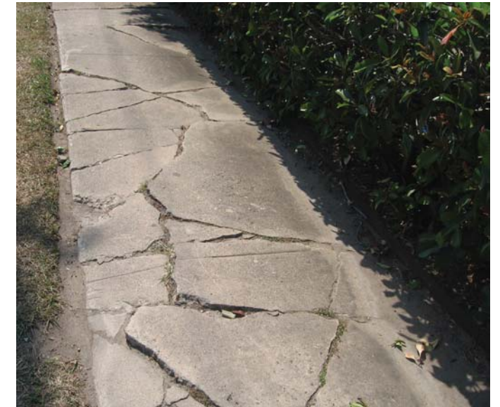
Photo 7-11, Segment 4A Westheimer between Huldy and Brun Sidewalk is cracked and has settled, creating tripping hazards.
