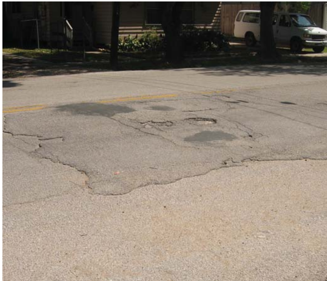
Photo 8-6, Segment 38B Fairview between Upas and Van Buren Sections of a previous patch have begun to come up and create pot holes.
