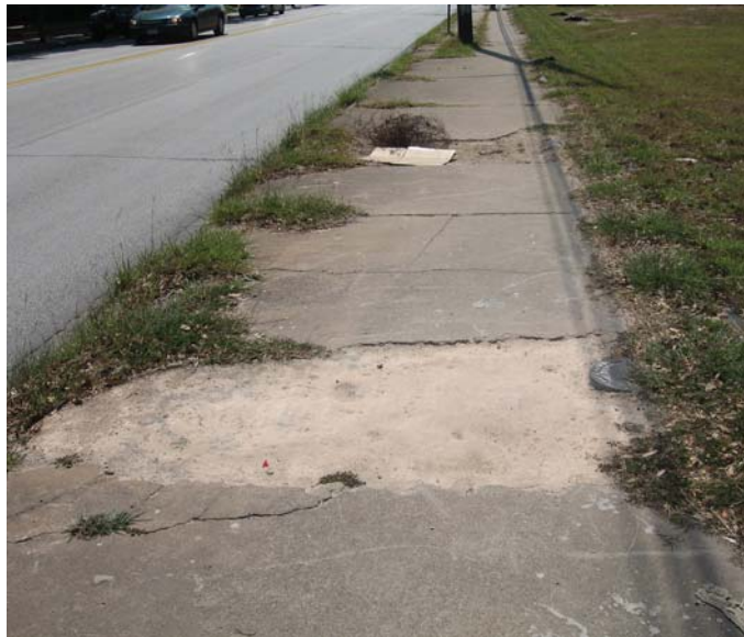
Photo 7-13, Segment 8A Westheimer between McDuffie and Hazard Missing sections of sidewalk periodically through out the block
