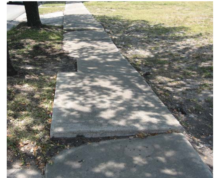
Photo 6-18, Segment 16A W. Alabama between Mandell and Mulberry Ground movement has caused whole sidewalk sections to shift, creating tripping hazards.
