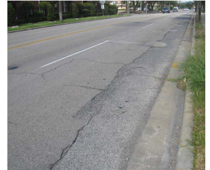
Photo 10-7, Segment 16B W. Dallas between Peveto and Joe Annie Road has settled near the curb.
