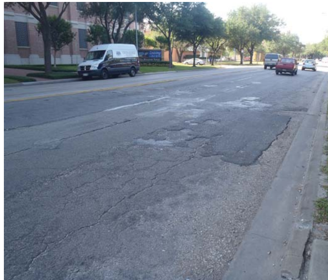
Photo 11-5, Segment 30A Montrose at between Banks and Milford There are multiple layers of asphalt in varying levels of disrepair that create an uneven riding surface.
