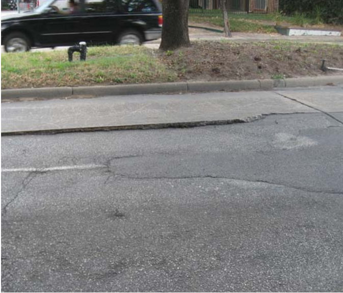
Photo 5-5, Segment 16B Richmond between Loretto and Yupon Pavement separation
