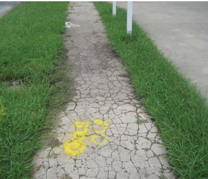
Photo 7-20, Segment 60A Westheimer between Whitney and Taft Severe cracks have formed in the sidewalk.
