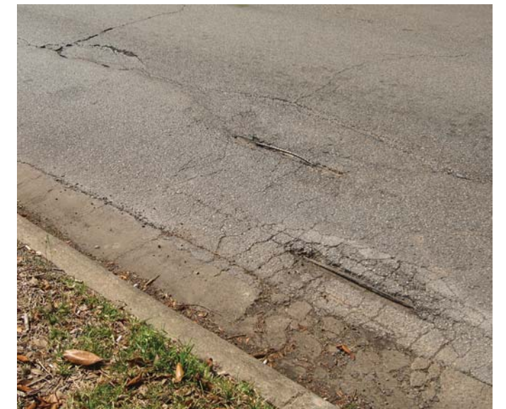
Photo 6-3, Segment 12B W. Alabama between Woodhead and Dunlavy Near the intersection with Dunlavy, there is exposed rebar.
