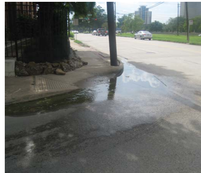
Photo 10-18 Segment 31 W. Dallas at Columbus Water accumulates at the bottom of the ramp
