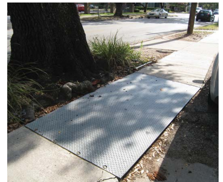
Photo 6-23, Segment 26A W. Alabama between Yoakum and Montrose This section is suitable for now, but should be monitored to make sure future tree root growth does not displace metal plate and create tripping hazard.
