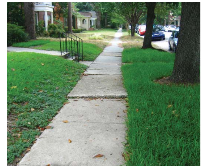
Photo 14-17, Segment 30A Dunlavy between Hawthorne and Harold Sidewalk sections have shifted, creating tripping hazards at joints.
