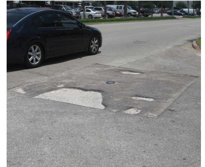
Photo 9-2, Segment 7 W. Gray at Driscoll Previous patch is coming up in sections, creating potholes and an uneven riding surface.
