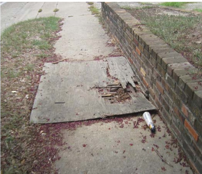
Photo 12-18, Segment 36B Waugh between Waughcrest and California Thin piece of plywood covers a hole in sidewalk.
