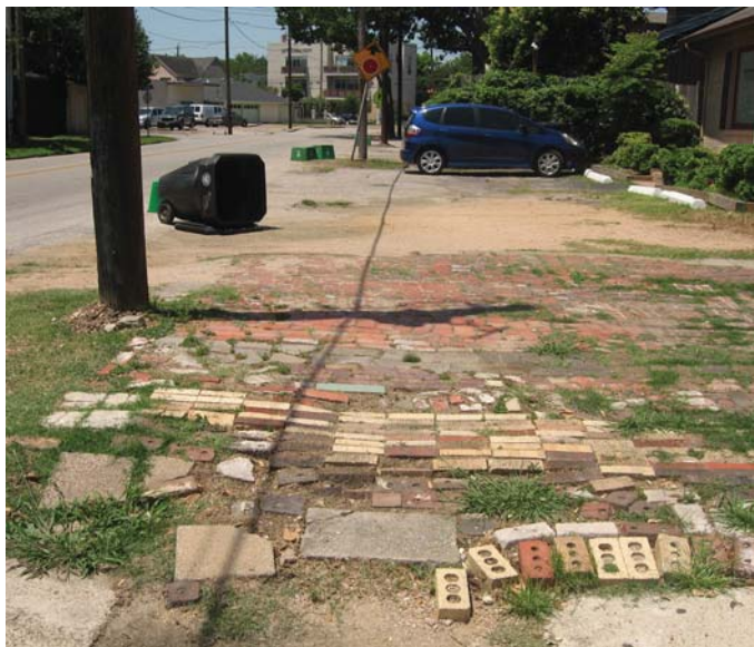
Photo 8-17, Segments 24A and 25 Fairview from Ralph to Mandell Uneven settling of the brick sidewalk have created a surface with many tripping hazards.
