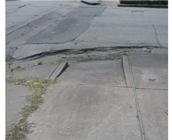
Photo 6-15, Segment 7 W. Alabama at Hazard Road resurfacing has made ramps difficult to traverse.
