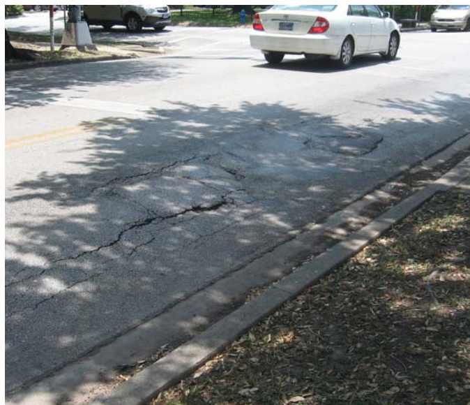
Photo 6-6, Segment 16A W. Alabama between Mandell and Mulberry There is a drop in the elevation of the pavement near the curb. The pavement is also cracking from the related stress.
